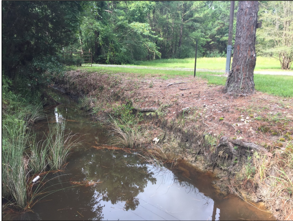
Figure 6.29 (1) Channel downstream of road crossing
