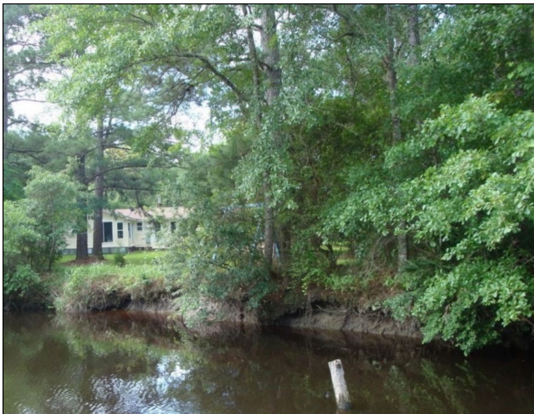
Figure 4.8 Eroding streambank along upper Bayou La Batre
