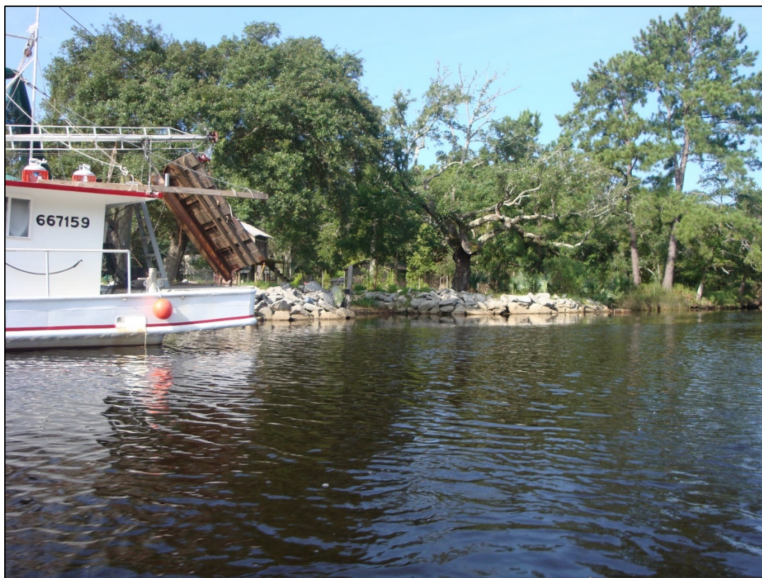
Figure 3.16 Revetment materials observed along shoreline of Bayou La Batre
