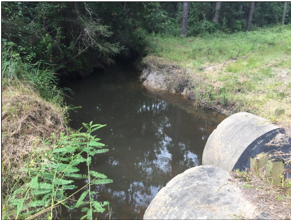
Figure 6.32 (2) Channel downstream of road crossing
