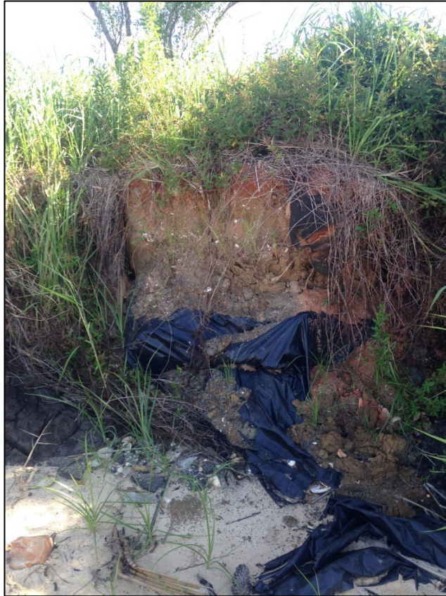
Figure 4.15 Evidence of filling of saltmarsh habitat at Lightning Point
