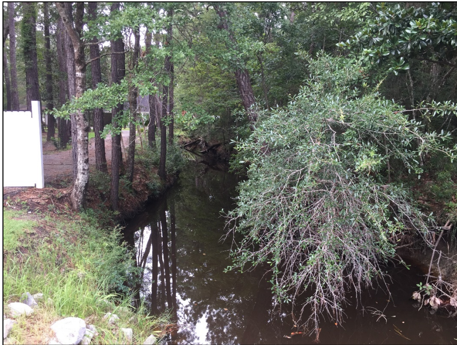
Figure 6.35 (3) Channel downstream of road crossing
