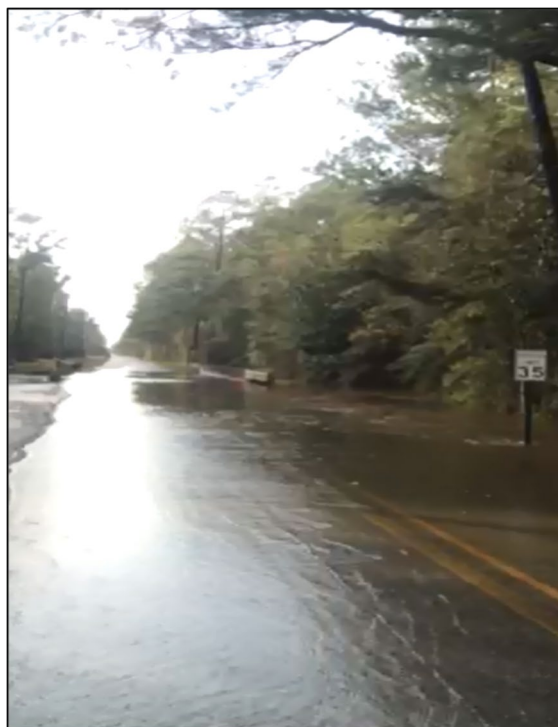
Figure 2.3 Davenport Street flooding (December 2015)
