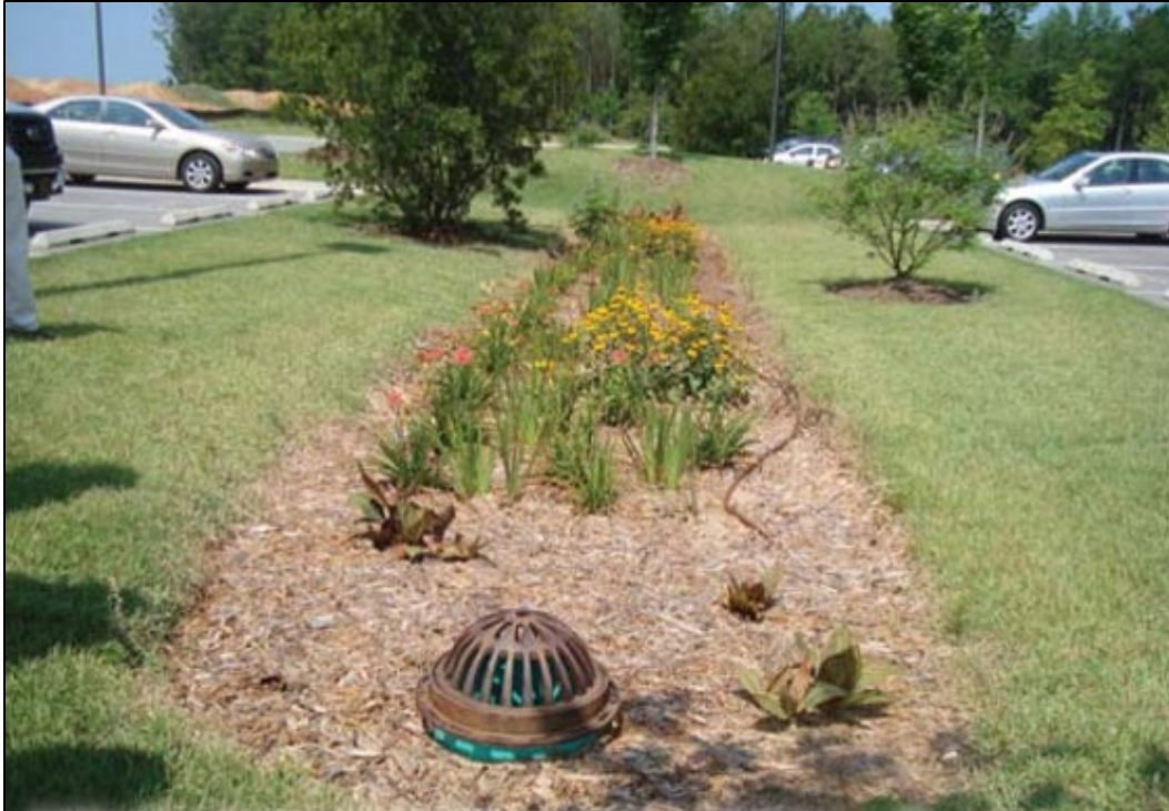
Figure 6.2 Example of bioretention swale in a parking area at Auburn Research Park; Auburn, AL (ADEM 2014)
