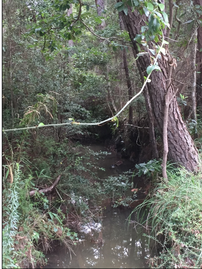
Figure 6.33 (2) Channel upstream of road crossing
