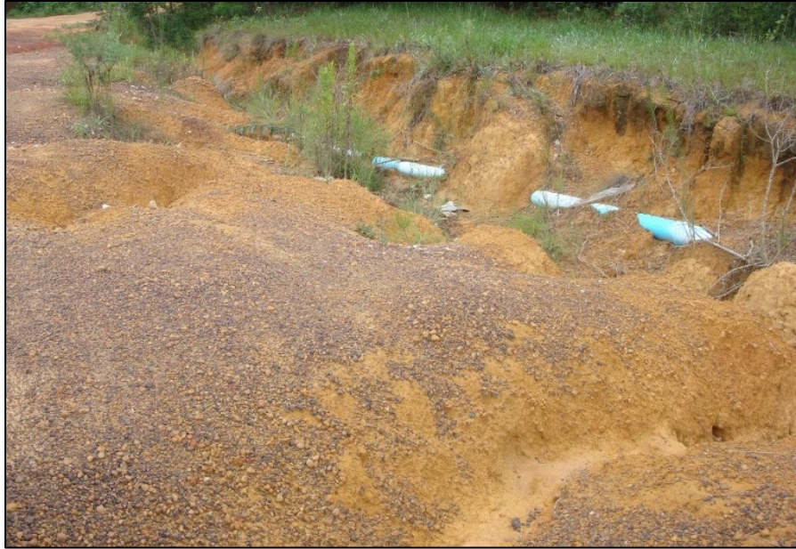
Figure 4. 1 Gullying and erosion in the upper Watershed from stormwater runoff
