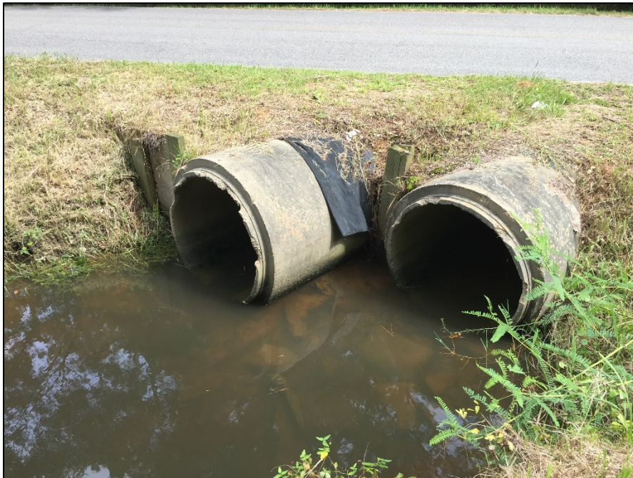
Figure 6.34 (2) Channel culvert crossing
