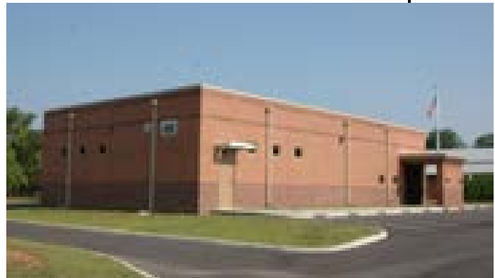
Figure 7.10: Chickasaw Community Shelter
