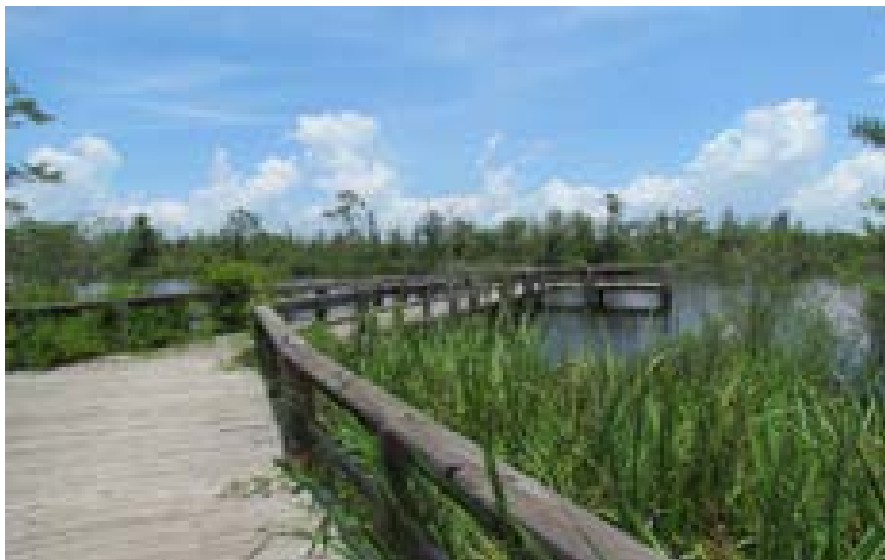
Figure 6.8: Boardwalk To One of Two Fishing Piers at Brooks Park
