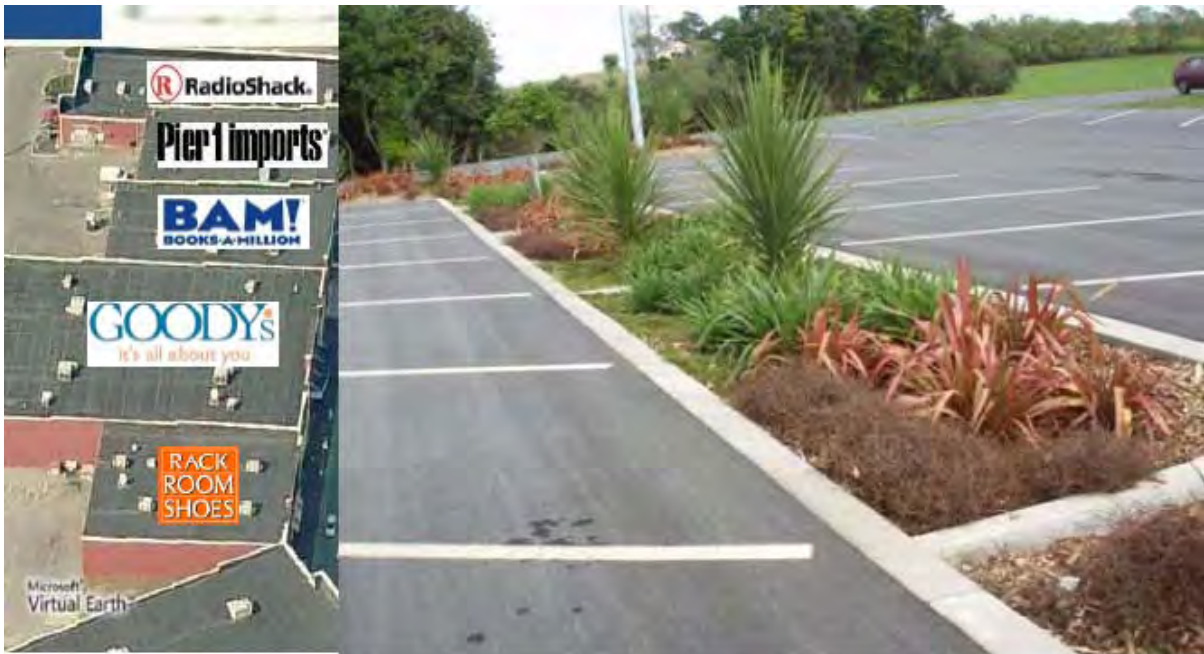
Figure 6-41. Example Application of Bioretention Area in Redevelopment Proposal for the Jubilee Square Shopping Center in Daphne. (Source: Presentation prepared by Goodwyn, Mills, and Cawood)
