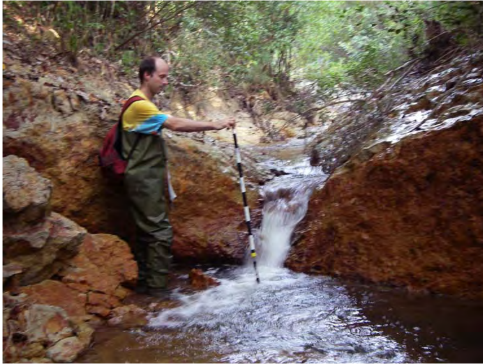
Figure 2-7. Head-cut through Erosion Resistant Streambed Materials on Tributary DA
