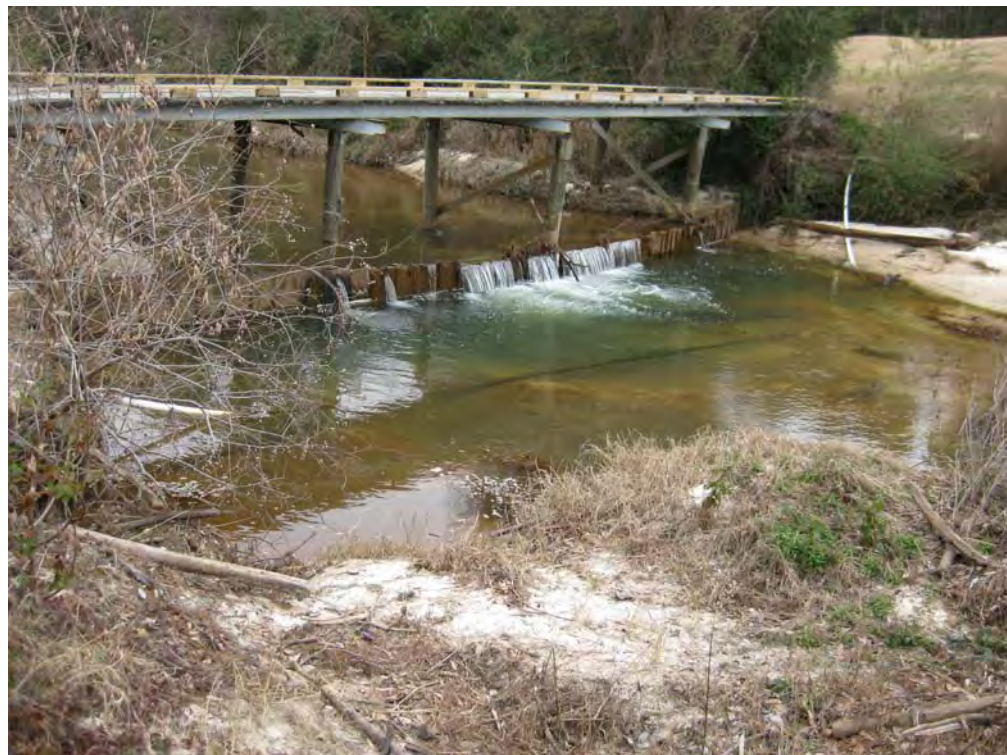
Figure 6-4. Sheetpile Grade Control Structure on Tiawasee Creek
