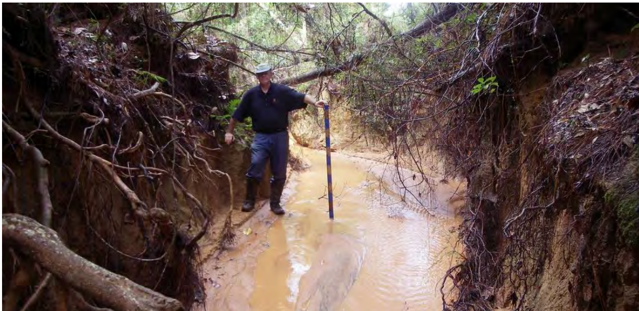
Figure 5-28. Incised reach of tributary JB undergoing bank mass wasting. Site JB6.
