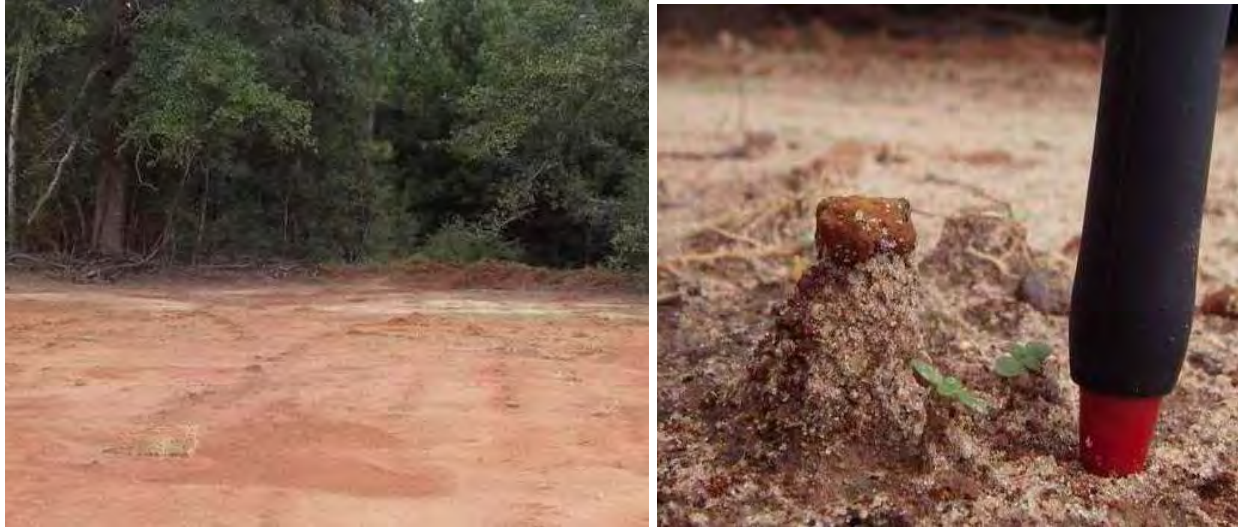
Figure 4-15. Construction site. Note 1/2 inch of soil loss marked by pedistalled pebble. Site U13.
