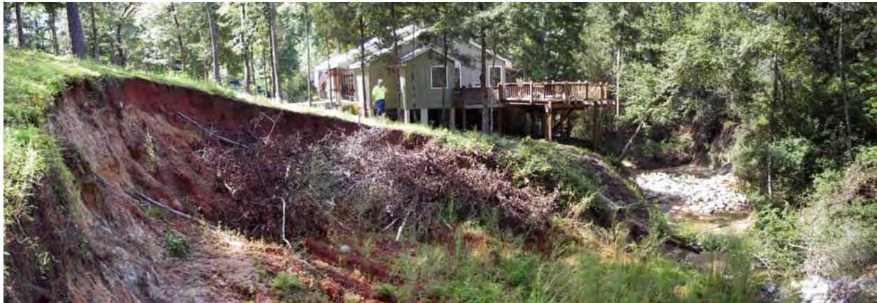
Figure 4-9. Recent mass wasting of streambank in Lake Forest. Site DA23a.
