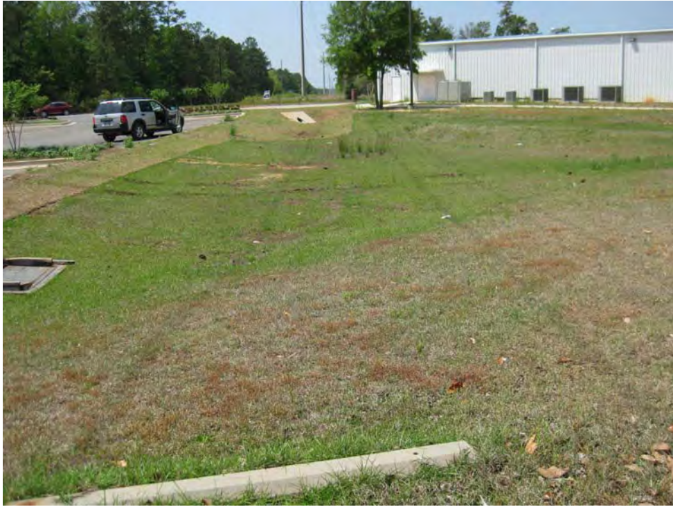
Figure 6-19. Possible Retrofit Location Waypoint 791 (Trojan Hall Fine Arts)
