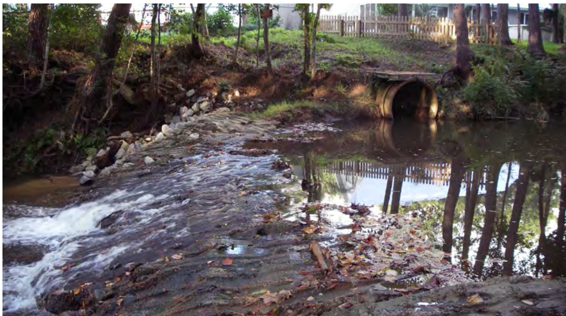
Figure 4-7. Existing Grade Control Structure on Tiawasee Creek Downstream of Tributary TB
