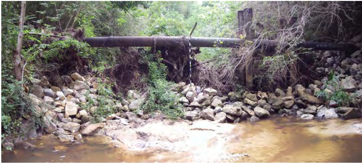
Figure 4-5. Pipeline Crossing on Tiawasee Creek Upstream of Confluence with Tributary TC Protected from Head-Cutting Induced Erosion
