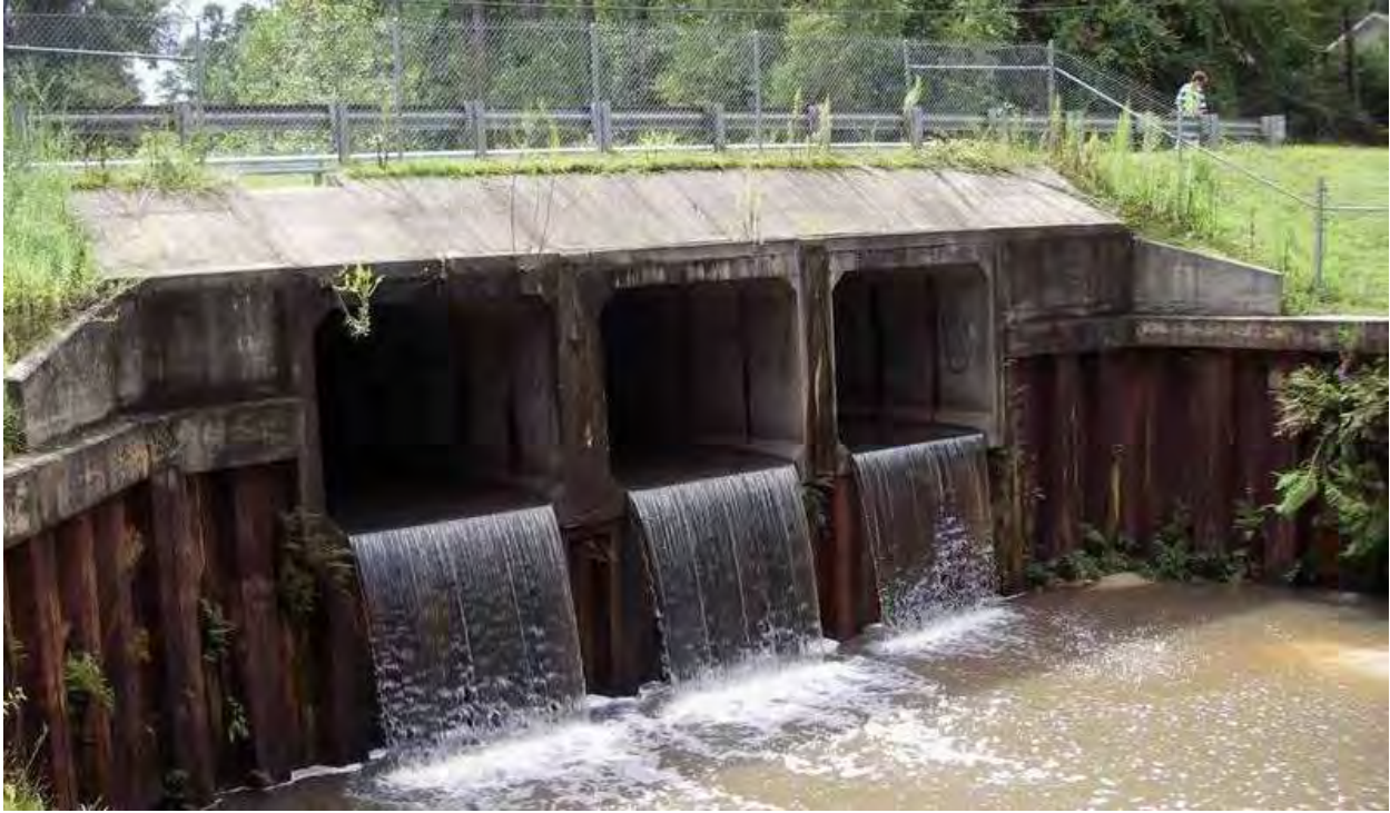
Figure 5-18. Concrete drop structure creates grade control below Greenwood Drive. Site TC1.
