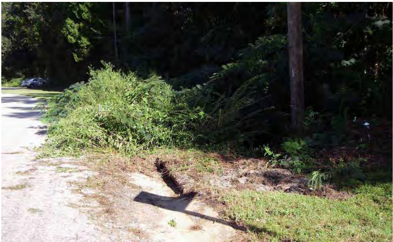
Figure 4-11. Four meter deep gully within 5 meters of road is totally obscured by vegetation. Site U37.
