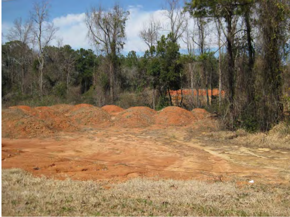
Figure 4-20. Unconfined Fill Dirt Not Yet Used for Construction
