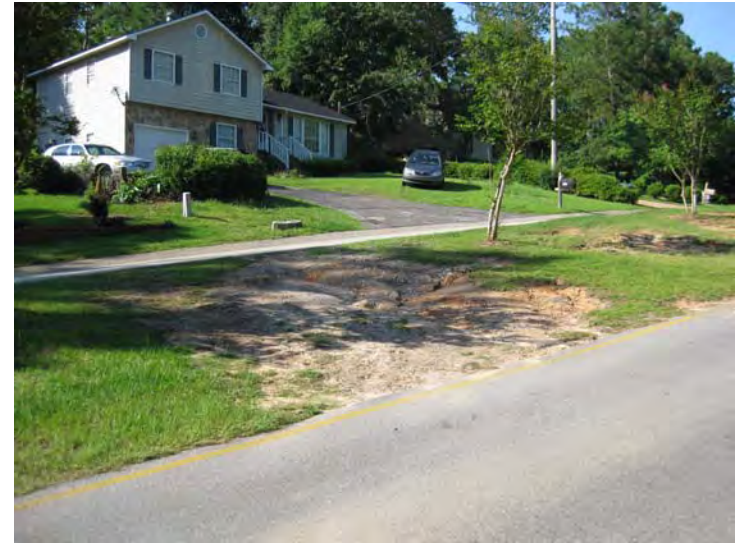
Figure 6-28. Examples of Erosion Problems Affecting the Road Medians of the Lake Forest Subdivision
