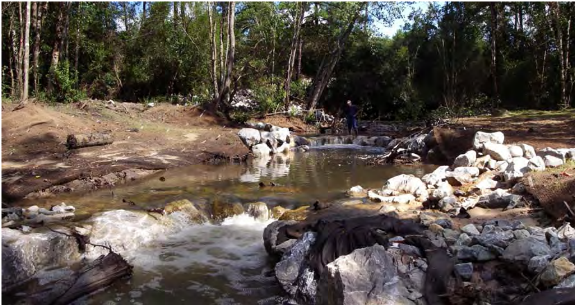
Figure 6-1. Stream Restoration Grade Control Structures on D'Olive Creek South of I-10
