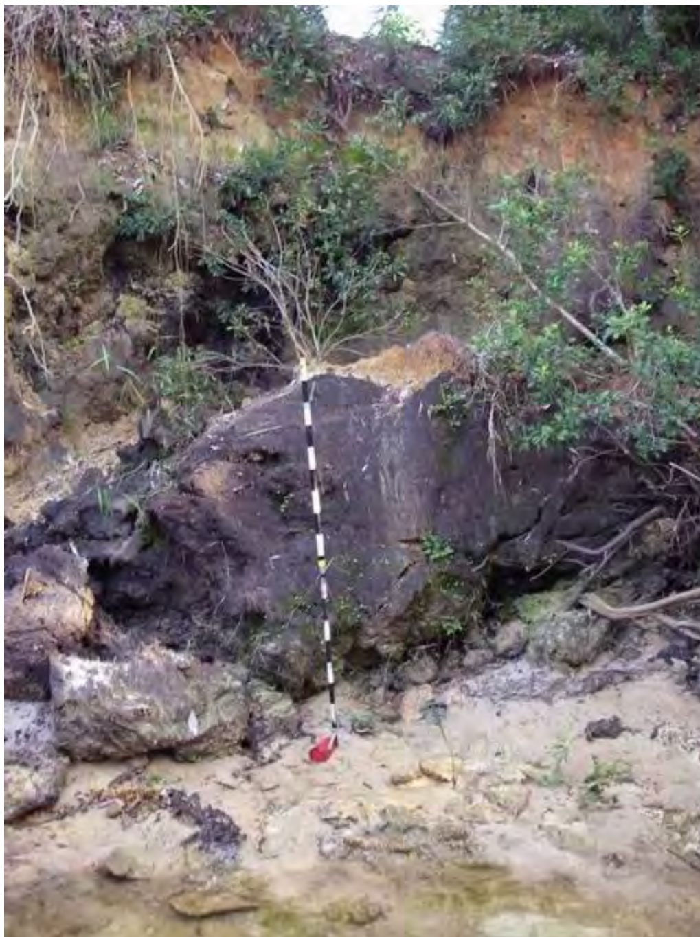
Figure 5-8. Mass wasting of streambank beneath power line crossing. Site DA36
