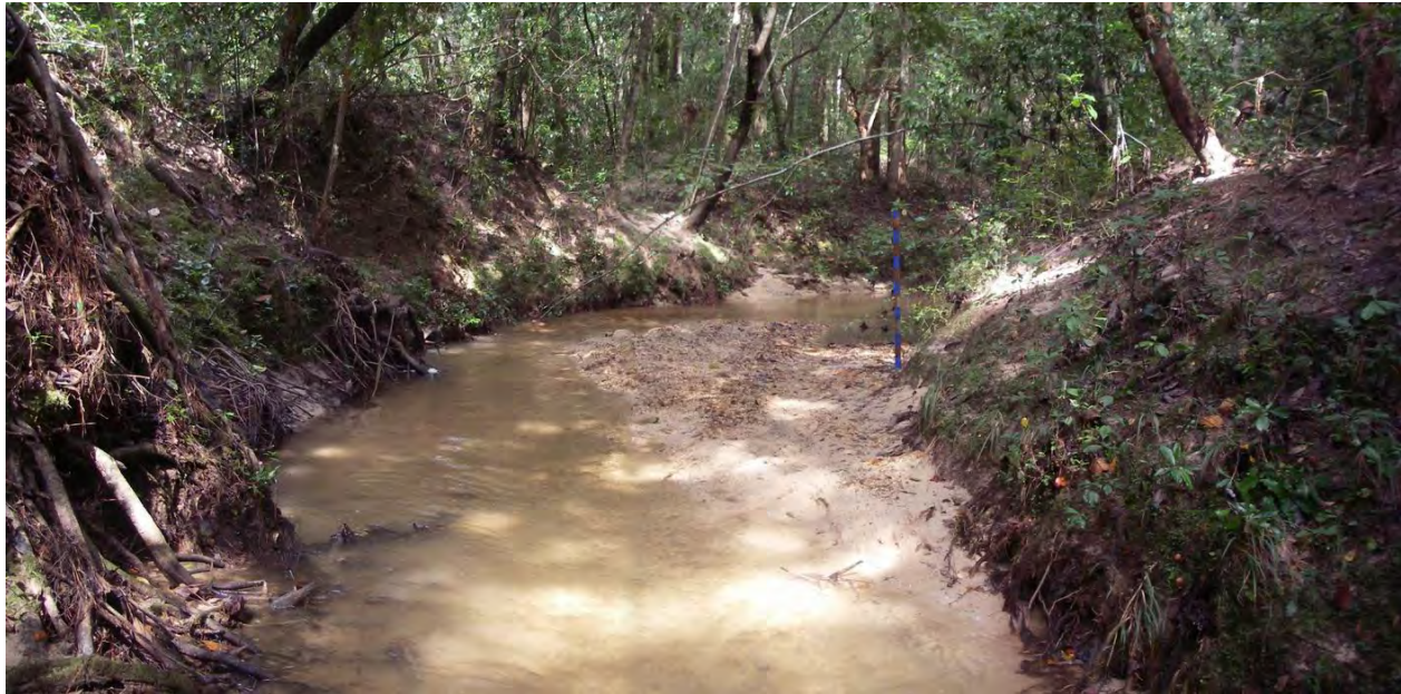
Figure 5-5. Reach impacted by both bank erosion and bed sedimentation. Site DA2.
