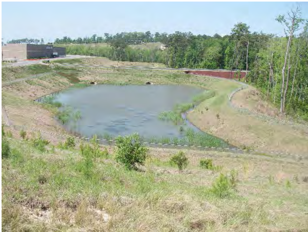
Figure 6-16. Detention Pond at Spanish Fort Town Center
