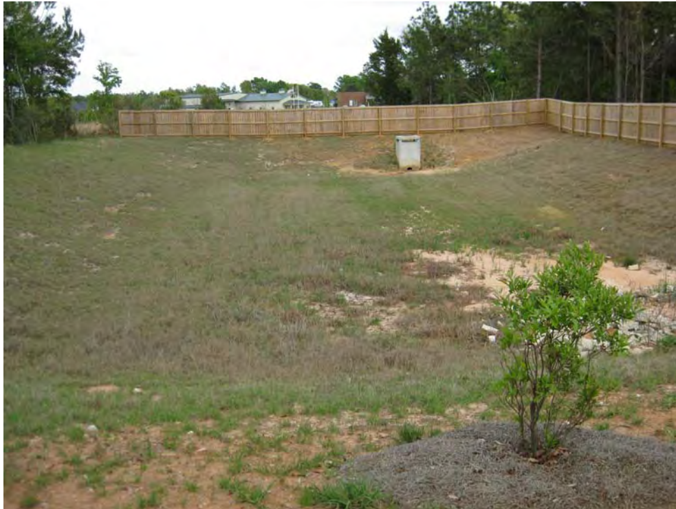
Figure 6-13. Detention Pond at Caroline Woods Subdivision
