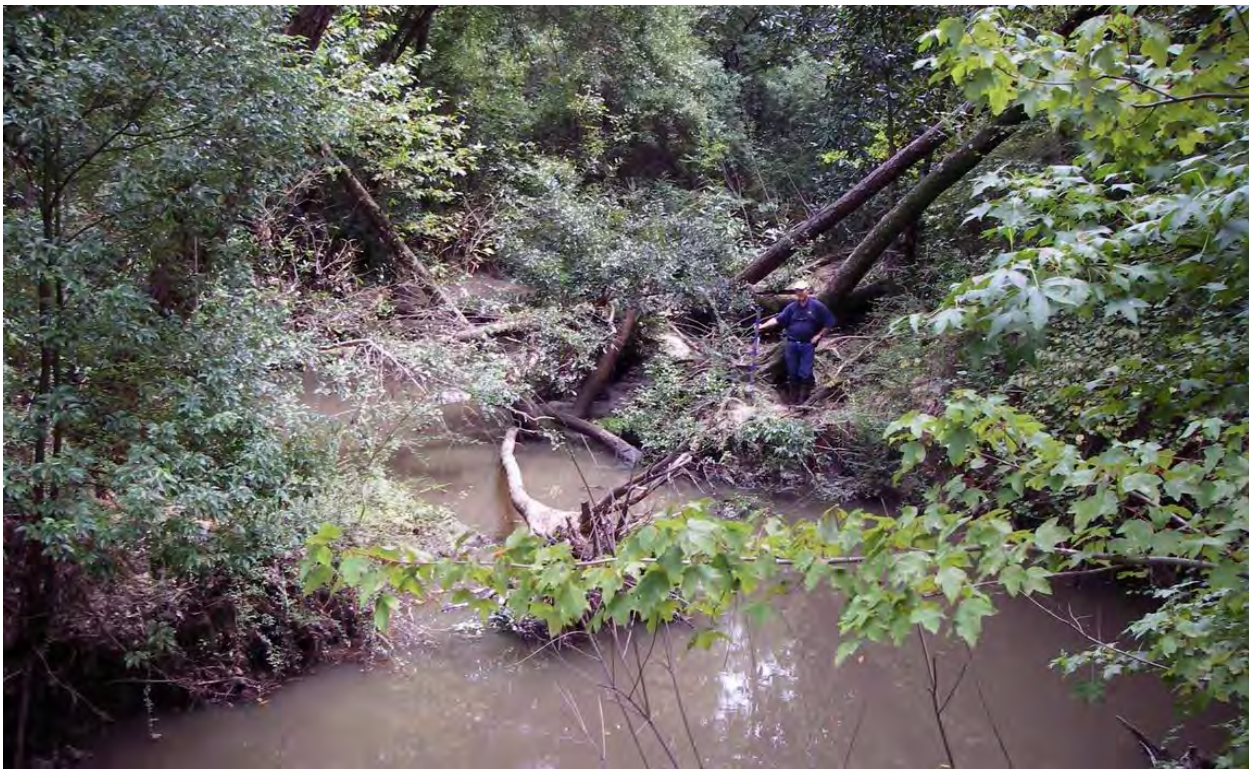
Figure 5-19. Person standing on rotational failure of high streambank with trees. Site TC2.
