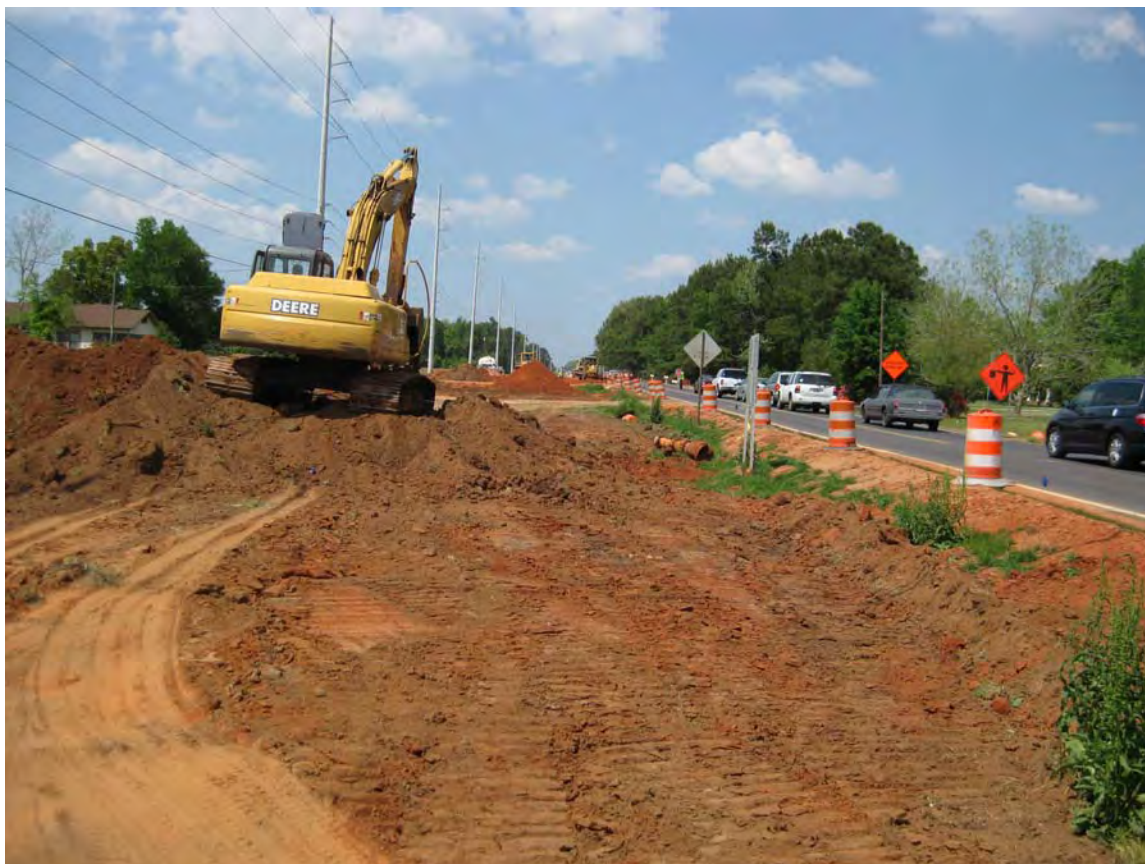
Figure 2-20. Widening in Progress of State Road 181
