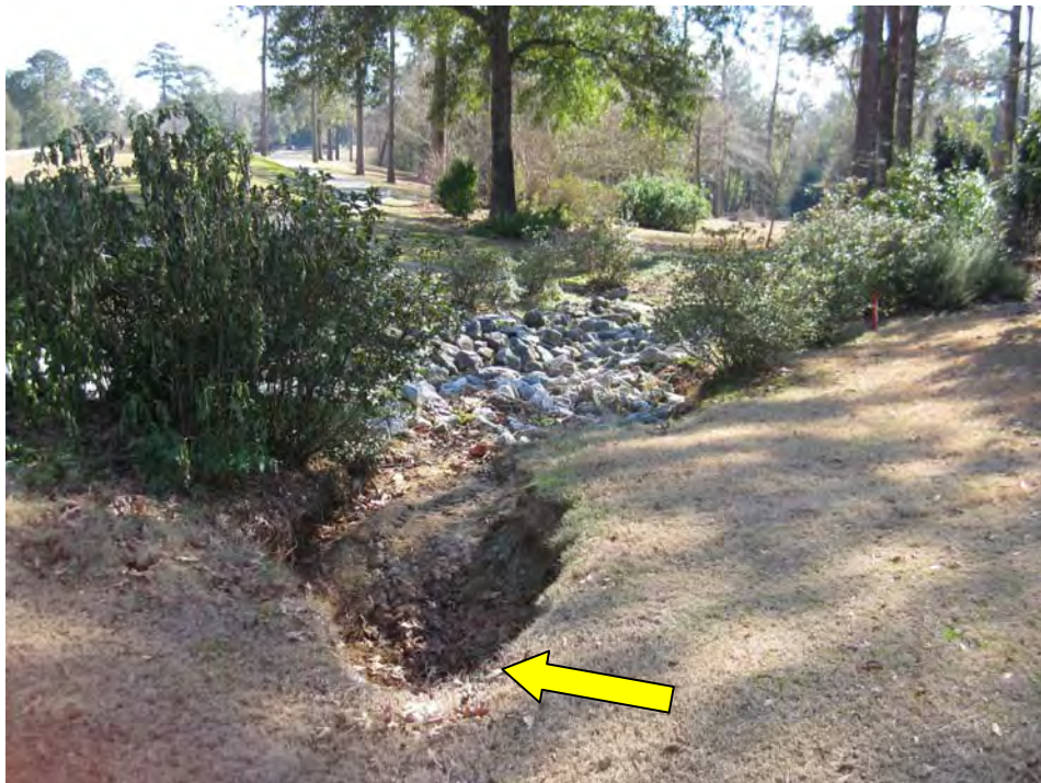
Figure 6-52. Example of Downslope Head-cutting Erosion from Stormwater Runoff Across Golf Course Fairway
