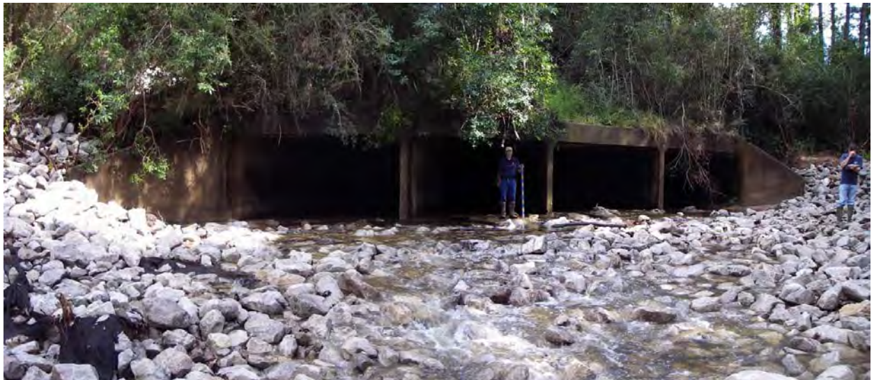
Figure 4-8. Scour repair below I-10 crossing of D'Olive Creek. Site D7.
