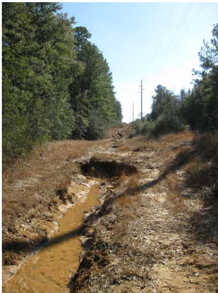
Figure 6-55. Typical Erosion Associated with Power Line Right-of-Ways
