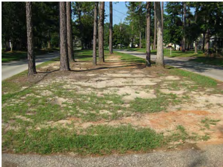
Figure 6-28. Examples of Erosion Problems Affecting the Road Medians of the Lake Forest Subdivision
