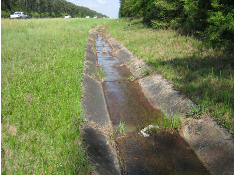
Figure 6-53. Existing Concrete-Line Drainage Ditch Along I-10
