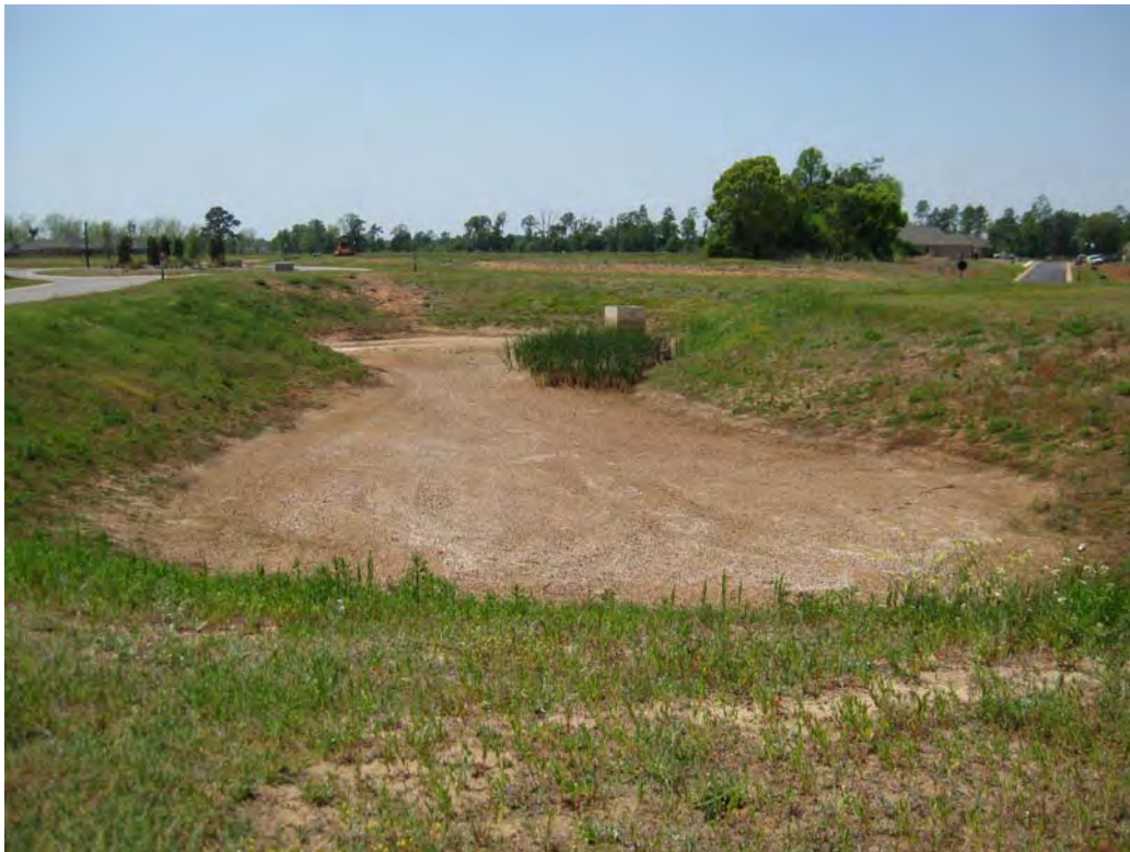
Figure 6-17. Detention Pond at French Settlement Subdivision (on two different occasions)
