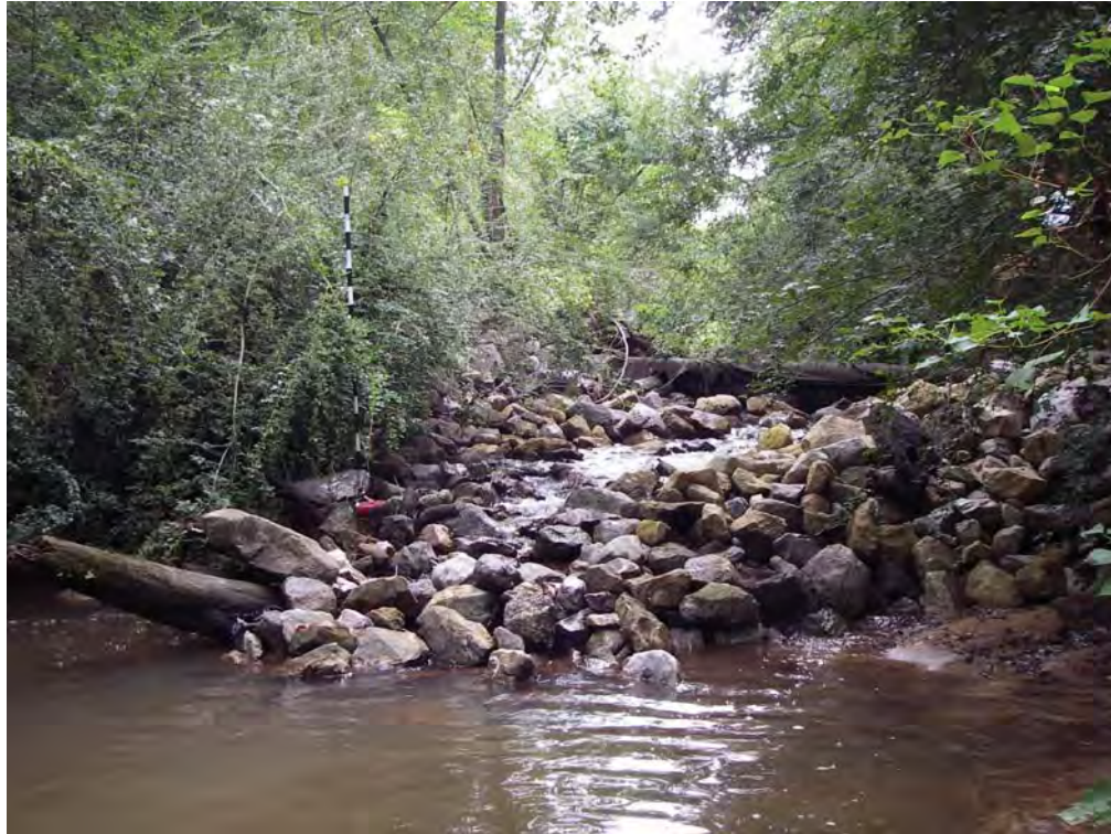
Figure 6-3. Riprap Grade Control Structure on Tiawasee Creek
