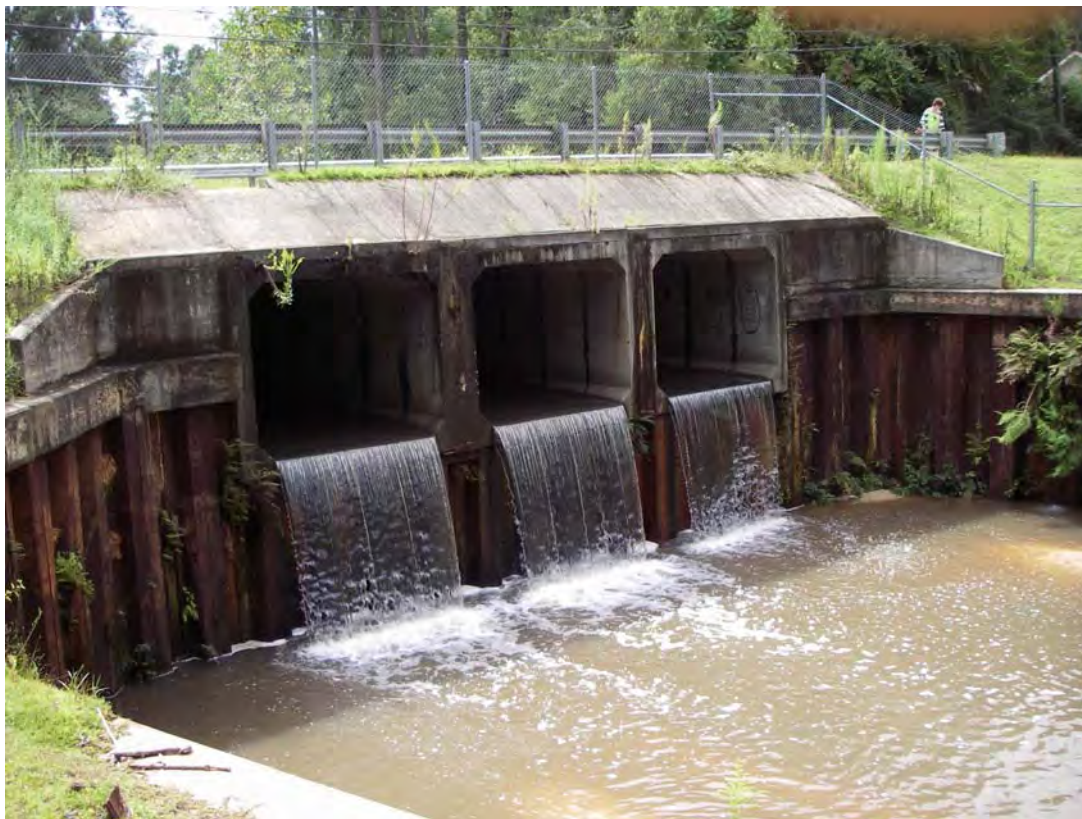
Figure 6-2. Grade Control at Tiawasee Creek Tributary (TC) Road Crossing
