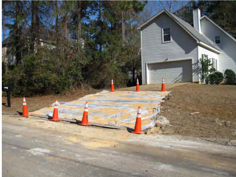
Figure 6-33. Driveway being replaced in the Lake Forest Subdivision
