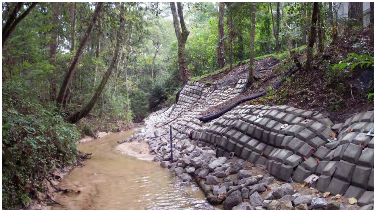
Figure 4-10. Bank protection along an incised reach of trib DA. Site DA9.
