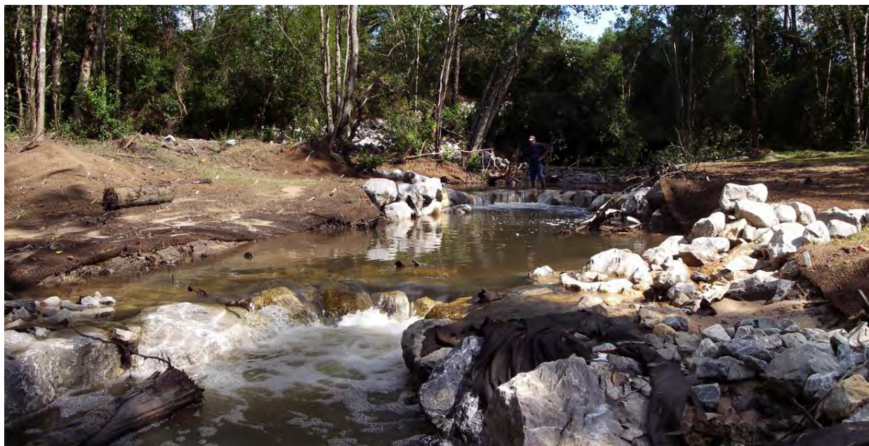
Figure 5-3. Restabilized reach below I-10. Site D6.
