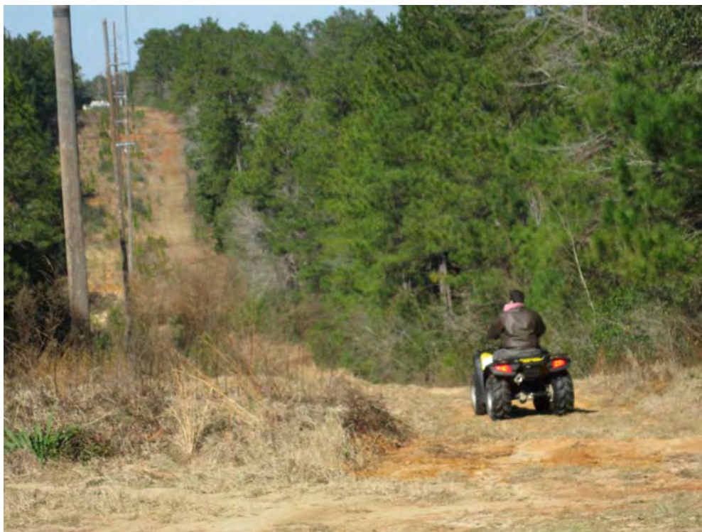
Figure 6-56. ATV Activity on Utility Right-of-Way.
