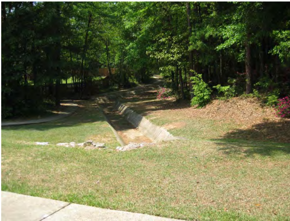
Figure 6-20. Possible Retrofit Location Waypoint 828 (Creekside Subdivision)
