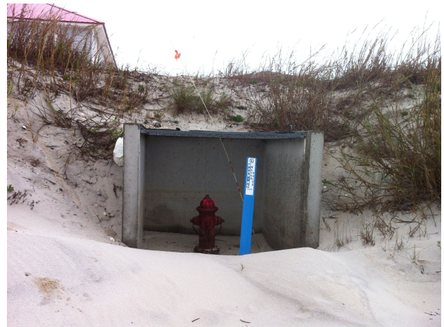
Photo: Protecting utilities on the West End Credit: T. Webler 2012
