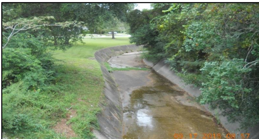
Figure 5.2.97: General view of Spencer Branch upstream from Cottage Hill Road
