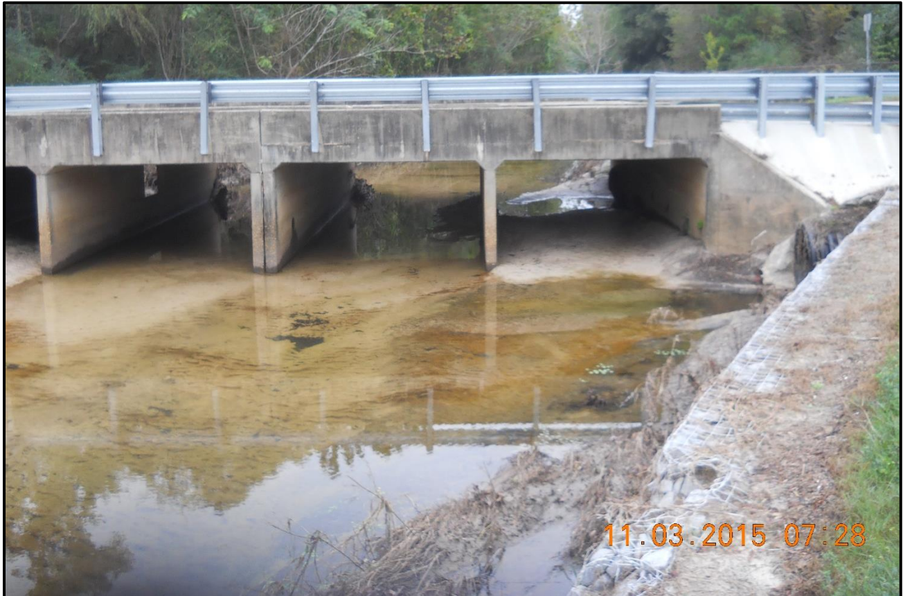
Figure 5.2.75: General view of sediment deposition (Spring Creek - at Halls Mill Road Crossing)
