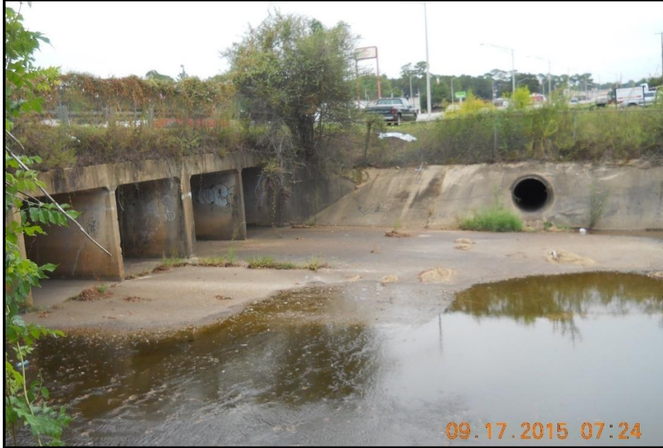
Figure 5.2.89: General view of Moore Creek (Moore Creek – Downstream of Government Boulevard)
