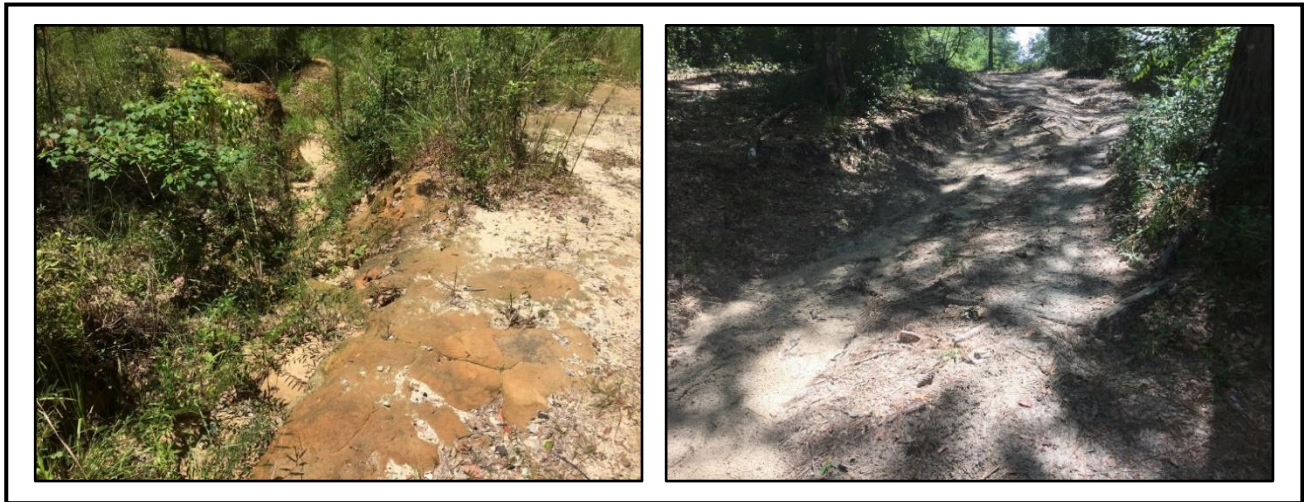
Figure 5.2.79: Examples of trespassing, ATV trails, and onsite erosion at Hippie Beach (Halls Mill Creek – N of Rangeline Road - adjacent to Cypress Business Park Drive)
