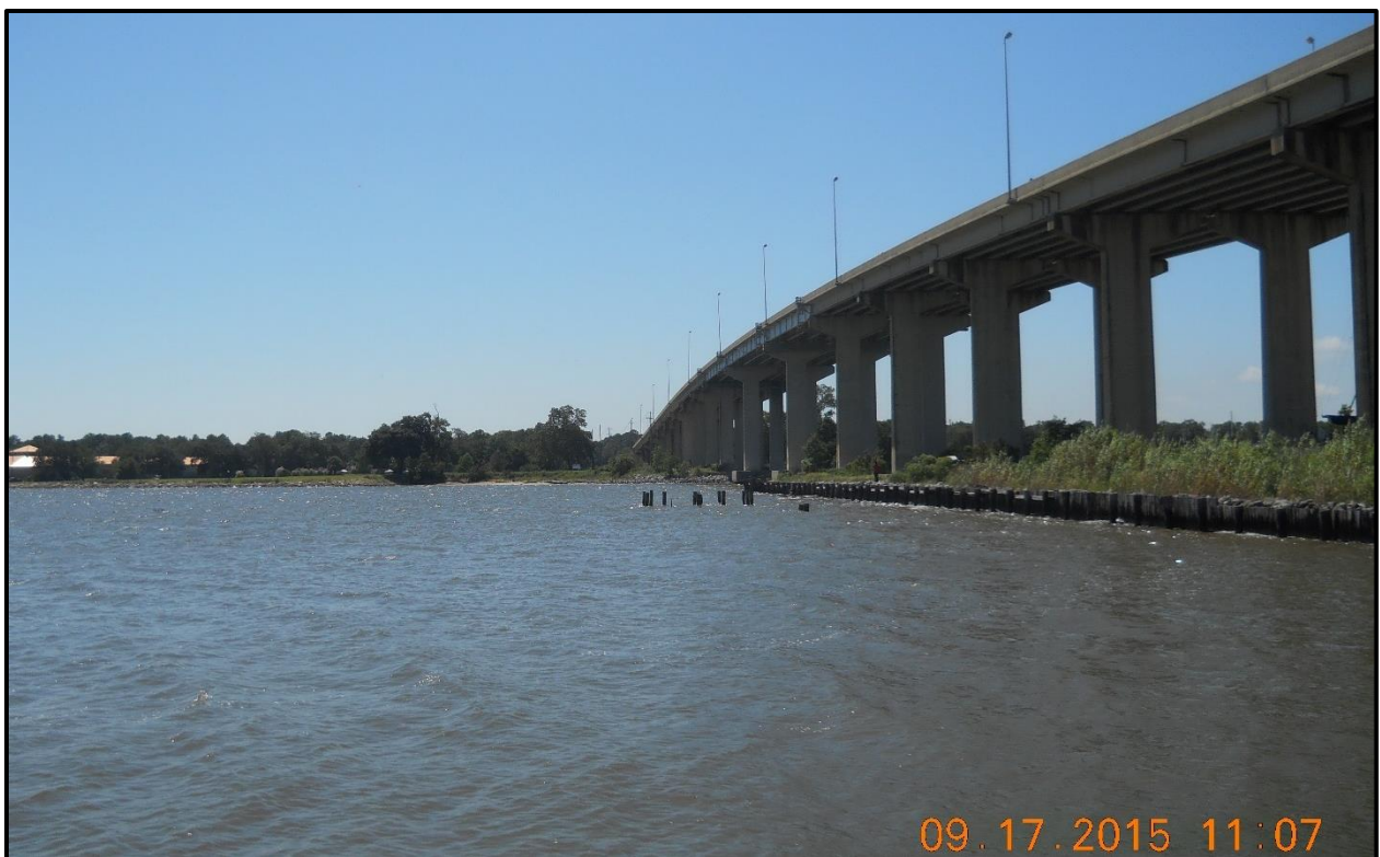
Figure 5.2.39: General view of lower Dog River near Dauphin Island Parkway
