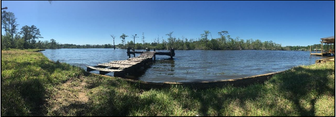
Figure 7.5.12: General example of an area suitable for a living shoreline along Halls Mill Creek
