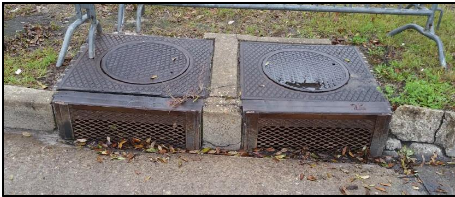
Figure 7.2.6: General example of catch basin screens (City of Mobile, 2016c)
