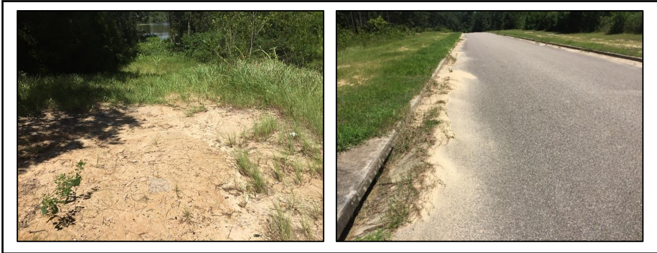
Figure 5.281: Examples of sediment migrating to the lowland areas (left) and sedimentation on street near stormwater drain (right) at Hippie Beach (Halls Mill Creek – N of Rangeline Road - adjacent to Cypress Business Park Drive)
