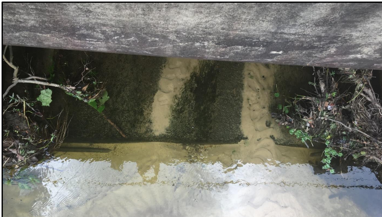
Figure 5.2.77: General view of box culvert (Spring Creek - at Halls Mill Road)
