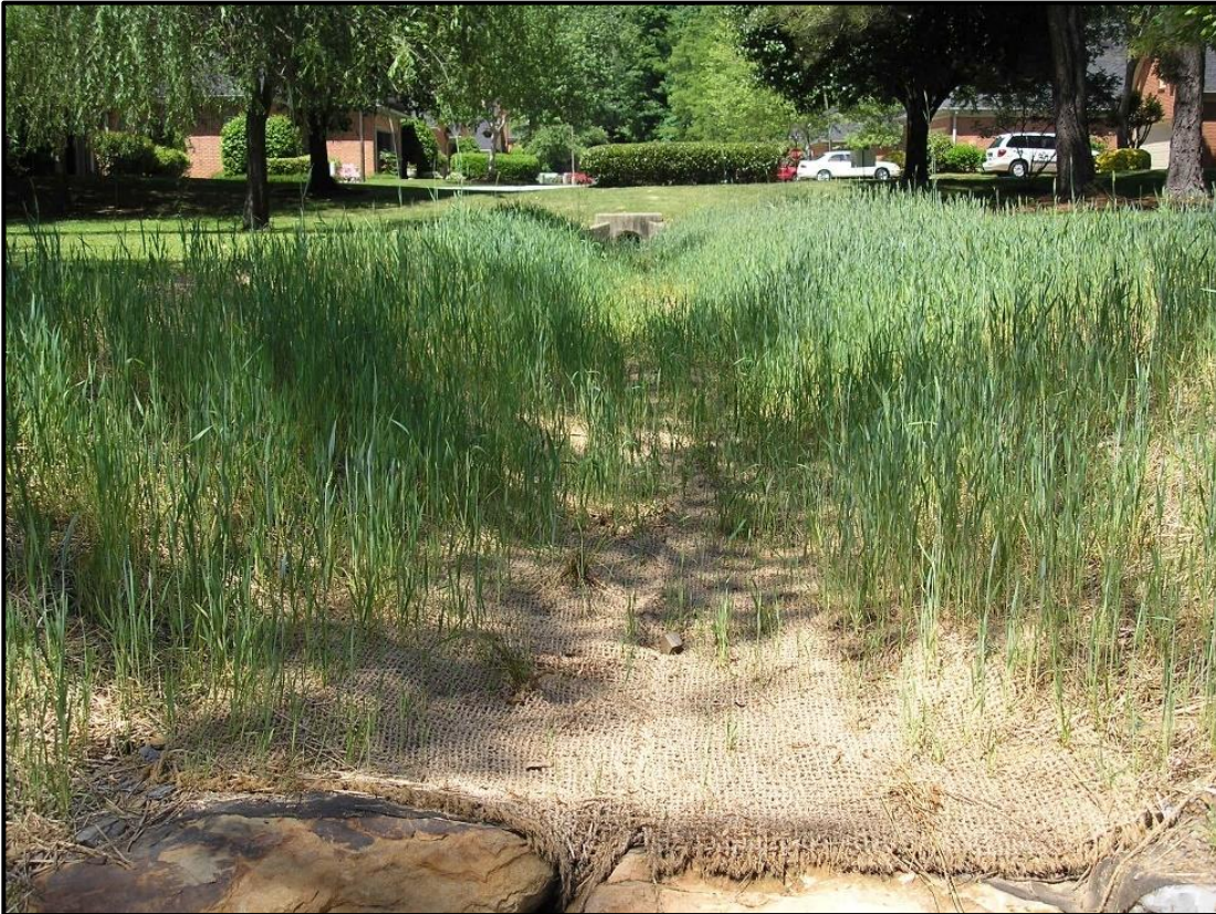
Figures 7.3.1: Vegetated bioretention swale application example
