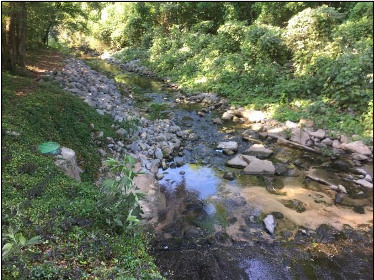
Figure 5.2.62: Riprap armoring on Spring Creek downstream from Maudelayne Drive North
