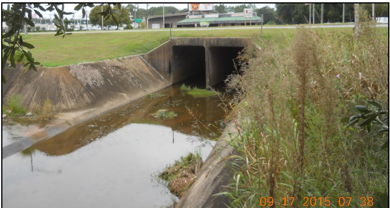
Figure 5.2.94: General view of East Bolton Branch at U.S. Highway 90 crossing
