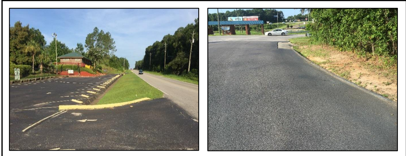
Figure 5.2.73: Examples of roadside drains (Spring Creek – near Girby Road)
