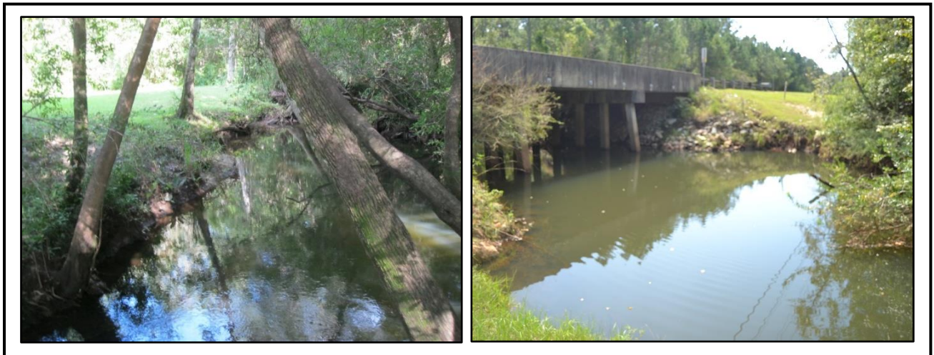
Figure 5.2.31: General views of Second Creek near its headwaters (left) and near Cody Road (right)
