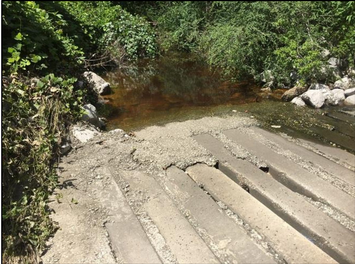
Figure 5.2.107: General view of the low-water crossing (Rattlesnake Bayou - Business Parkway)
