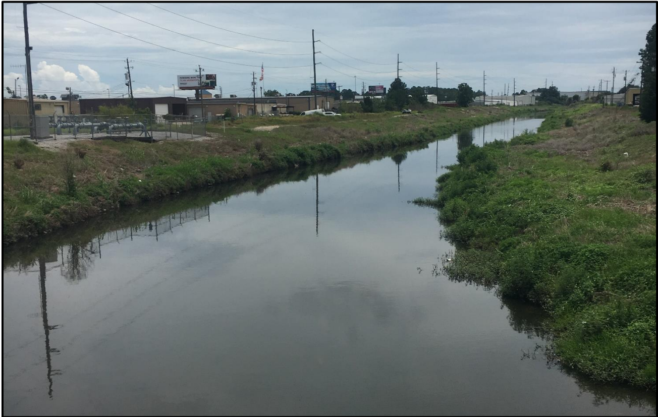
Figure 5.2.95: General view of Montlimar Canal downstream of Cottage Hill Road crossing
