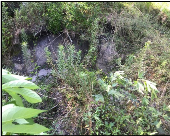
Figure 5.2.56: Example of eroding Banks (Spring Creek – Timberland Drive to Longleaf Drive)
