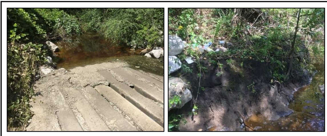
Figure 7.5.8: I-10 ramp to Motel Court potential restoration area
