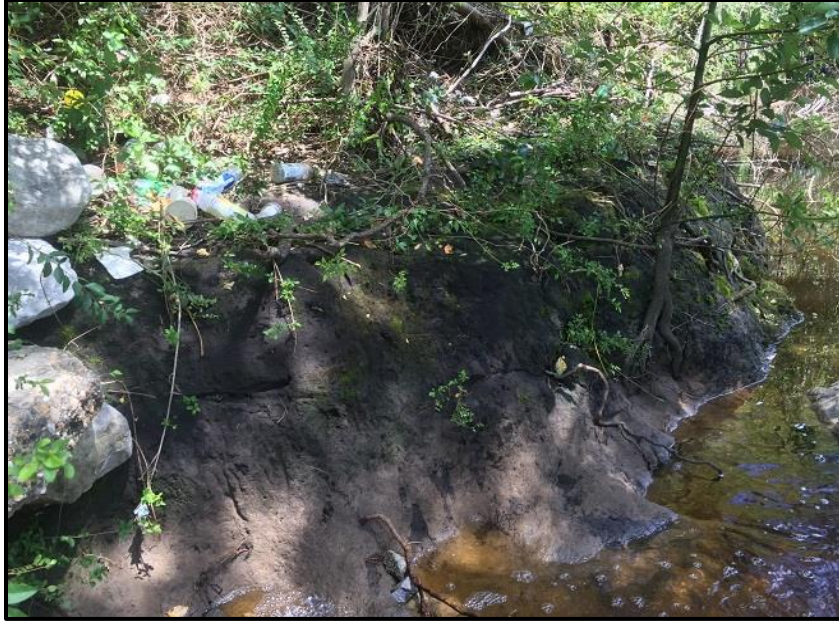
Figure 5.2.108: General view of eroding banks (Rattlesnake Bayou - Business Parkway)
