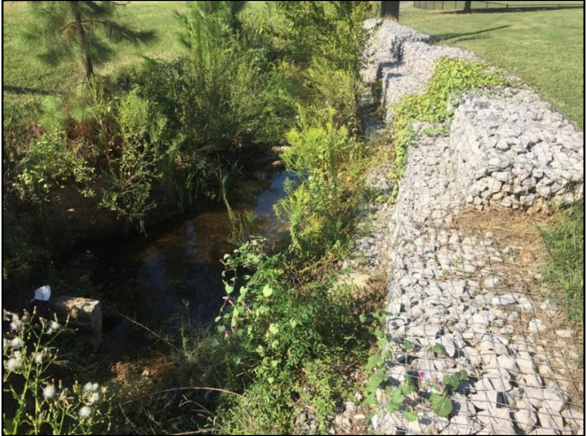
Figure 5.2.45: Example of gabion structures being used along a streambank in the greater Dog River Watershed
