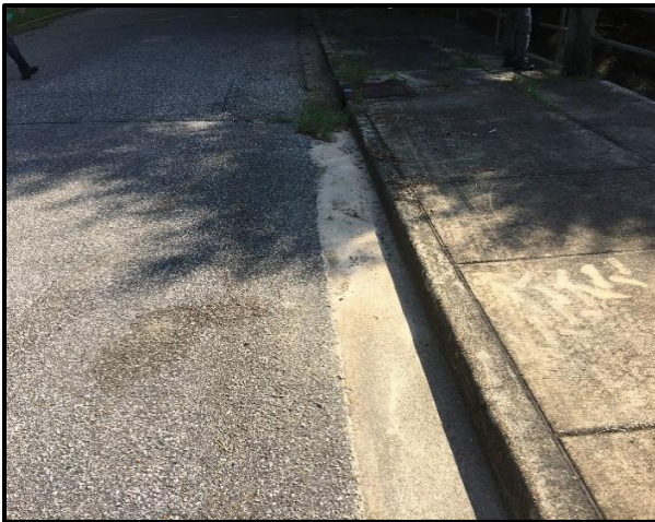
Figure 5.2.58: Sediment deposition on curb on Timberlane Drive drain (Spring Creek – Timberland Drive to Longleaf Drive)
