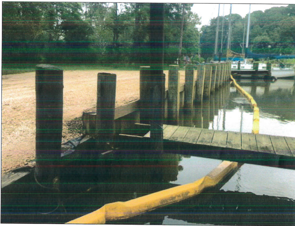
Pictured: City stormwater project - bulkhead at Fly Creek (Fairhope Docks marina)
