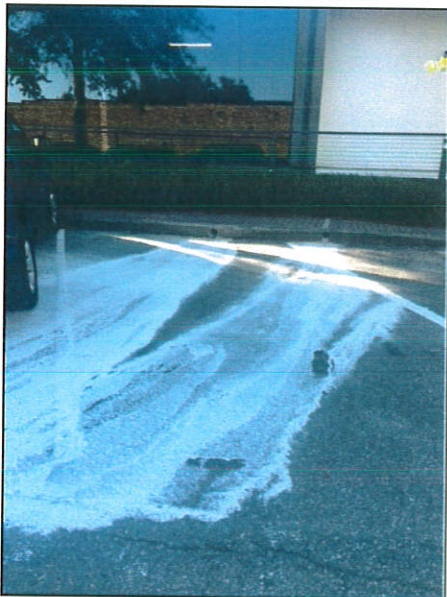
Pictured: Dry wall rinse water, potential illicit discharge, October 2018 reported by Public Works staff
