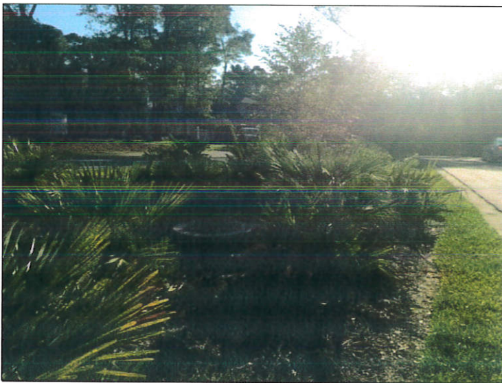
Pictured: LID stormwater facility in Pointe Place II
