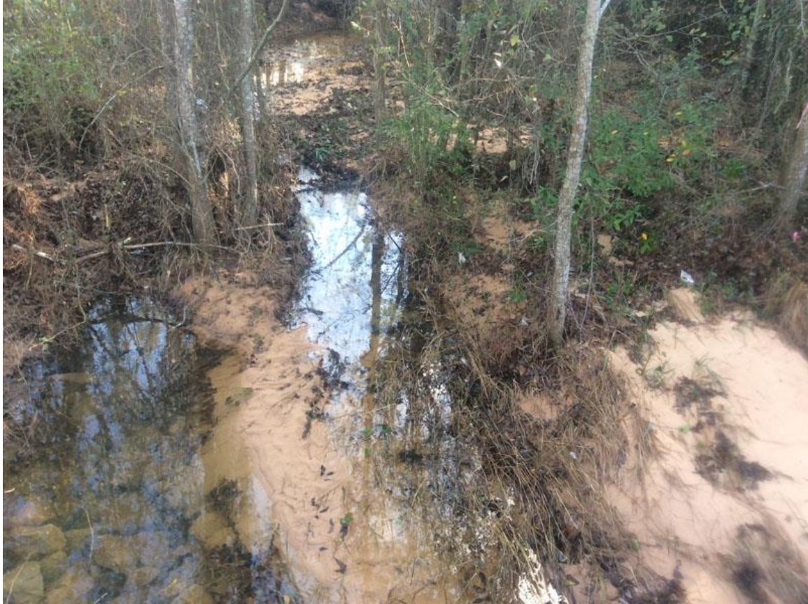
Figure 3.44 Degraded and Silted Drainageway Wetlands near the Intersection of CR 32 and CR 9
