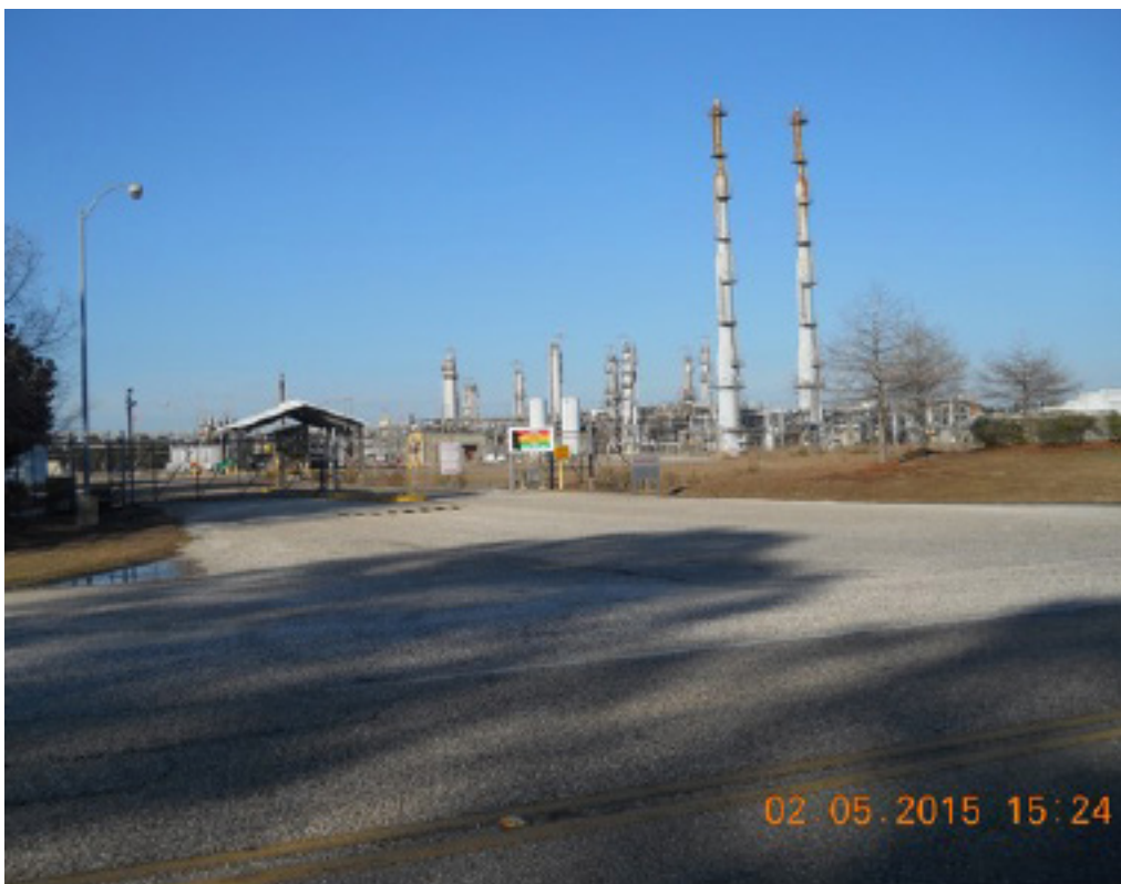
Figure 3.45: Industry along Deakle Road in Sub-watershed 6
