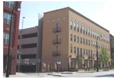
Parking deck with liner Building along street
