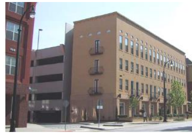
Parking deck with liner Building along street
