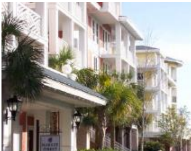
Buildings with high percentage of Fenestration and balconies on upper floors
