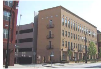
Parking deck with liner Building along street
