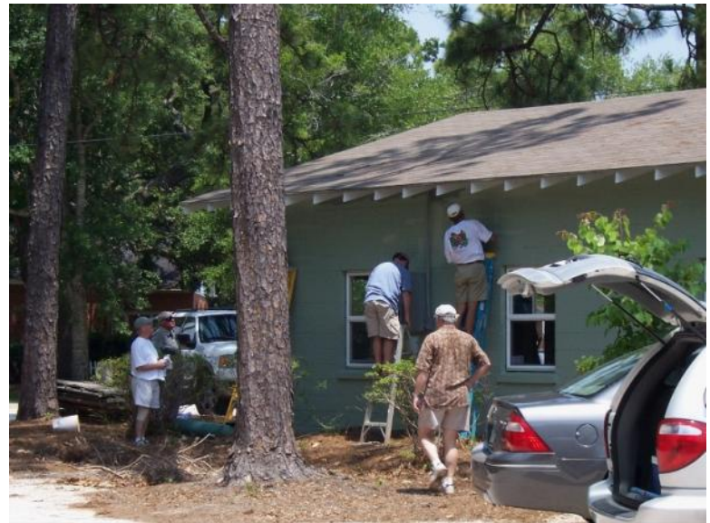
Figure 4-2: Resident Volunteers Renovating Town Hall Source: Town of Magnolia Springs
