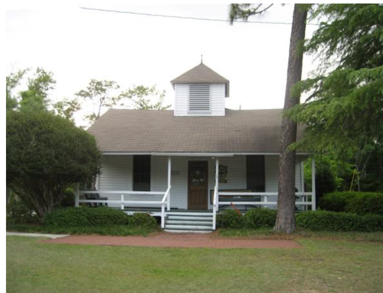
Figure 4-4: Magnolia Springs Community Association Building Source: Gould Evans
