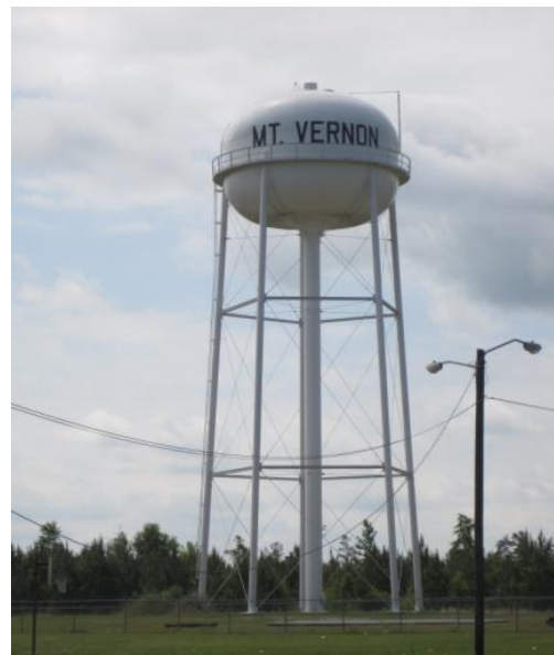
Figure 24 Mount Vernon Water Tower
