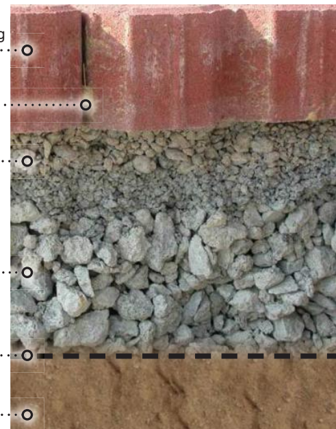
Section through PICP
