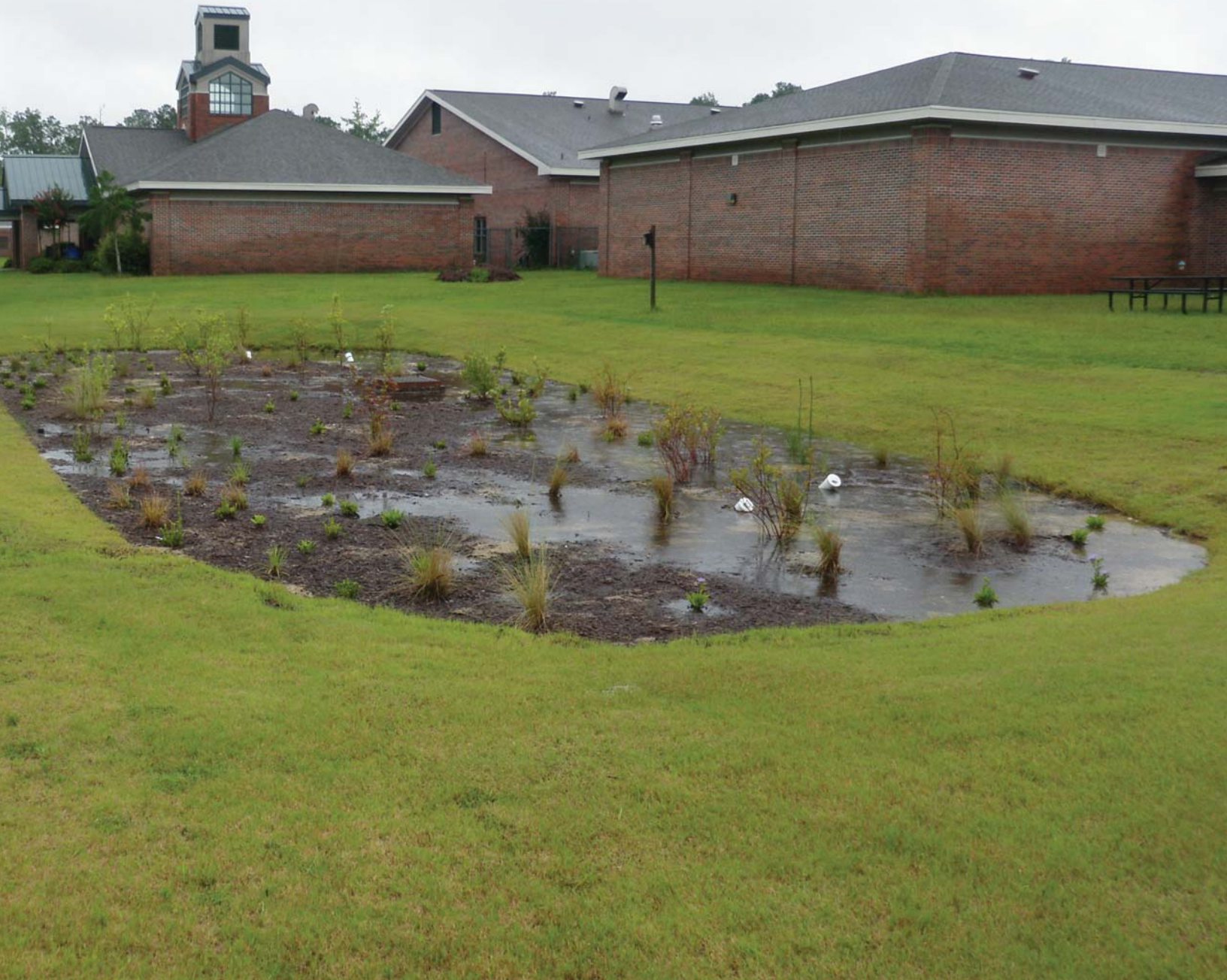
Bioretention cell 3 months post installation, East Smiths Station Elementary School; Smiths Station, AL
