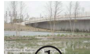
Synonyms: Bioretention basin
