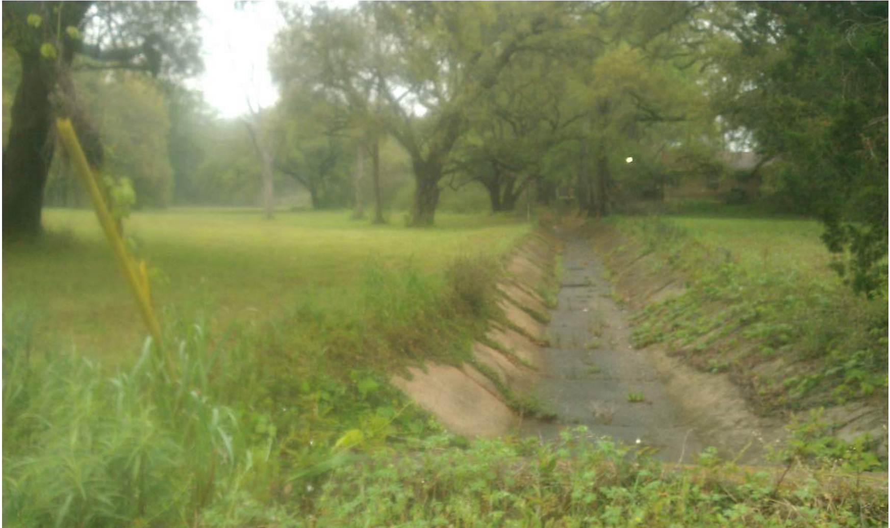
Figure 3-8 Concrete lined channel prohibits infiltration increasing stormwater runoff volumes and pollutant loads to Three Mile Creek, degrading water quality and habitat (Location: Three Mile Creek downstream of Cody Road, uppermost segment of the stream).
