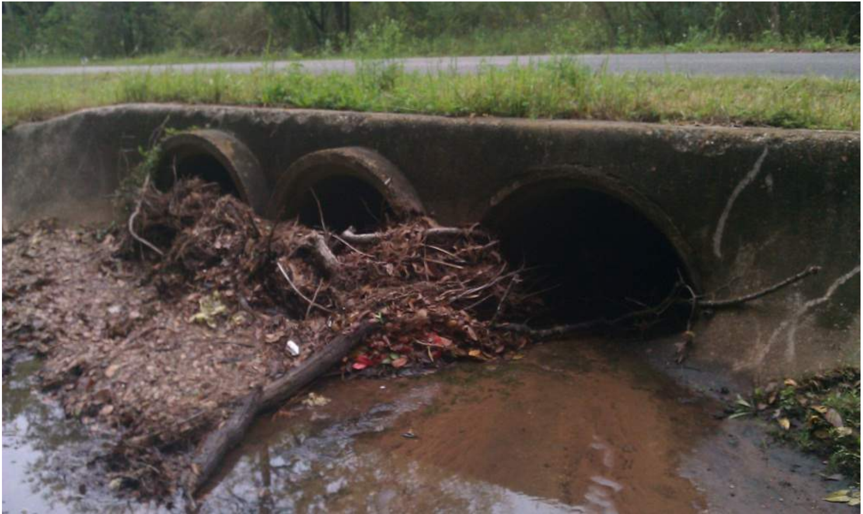
Figure 3-21 Unmaintained channels accumulate organic debris that rots placing an additional oxygen demand on the creek and degrading surface water quality and habitat (Location Twelve Mile Creek at Fontaine Drive).
