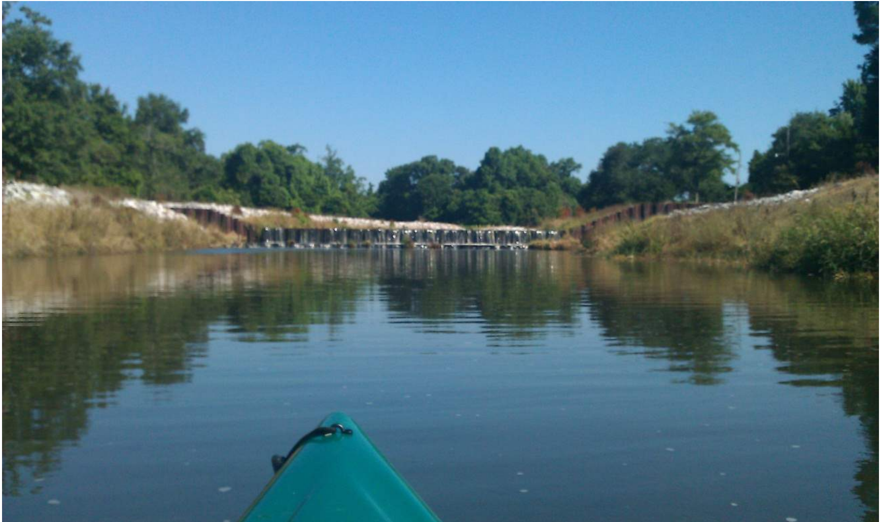
Figure 3-6 Deepening of the channel from the USACE project disconnected Three Mile Creek from its floodplain (Location: Three Mile Creek most upstream USACE weir upstream of I-65).
