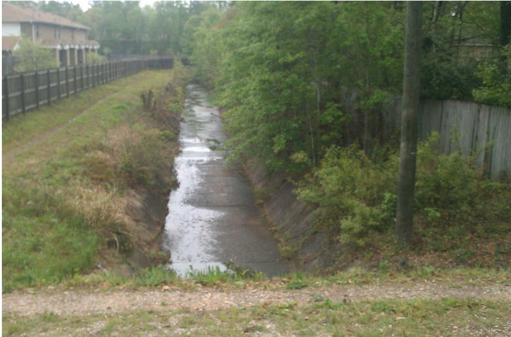
Figure 3-9 Concrete lined channel with mowed maintenance path on one side interrupting riparian corridor (Location: Twelve Mile Creek downstream of Hillcrest Road)
