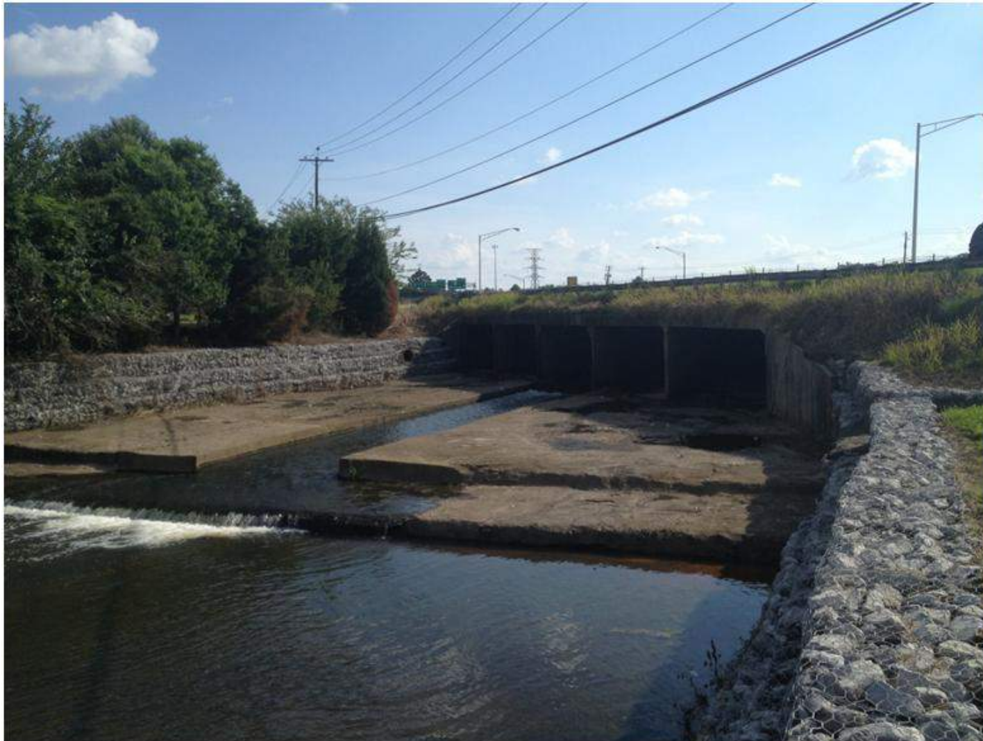
Figure 3-33 Gabion baskets create nearly vertical walls downstream of I-65; these prevent access to the creek and are a significant challenge during portage.
