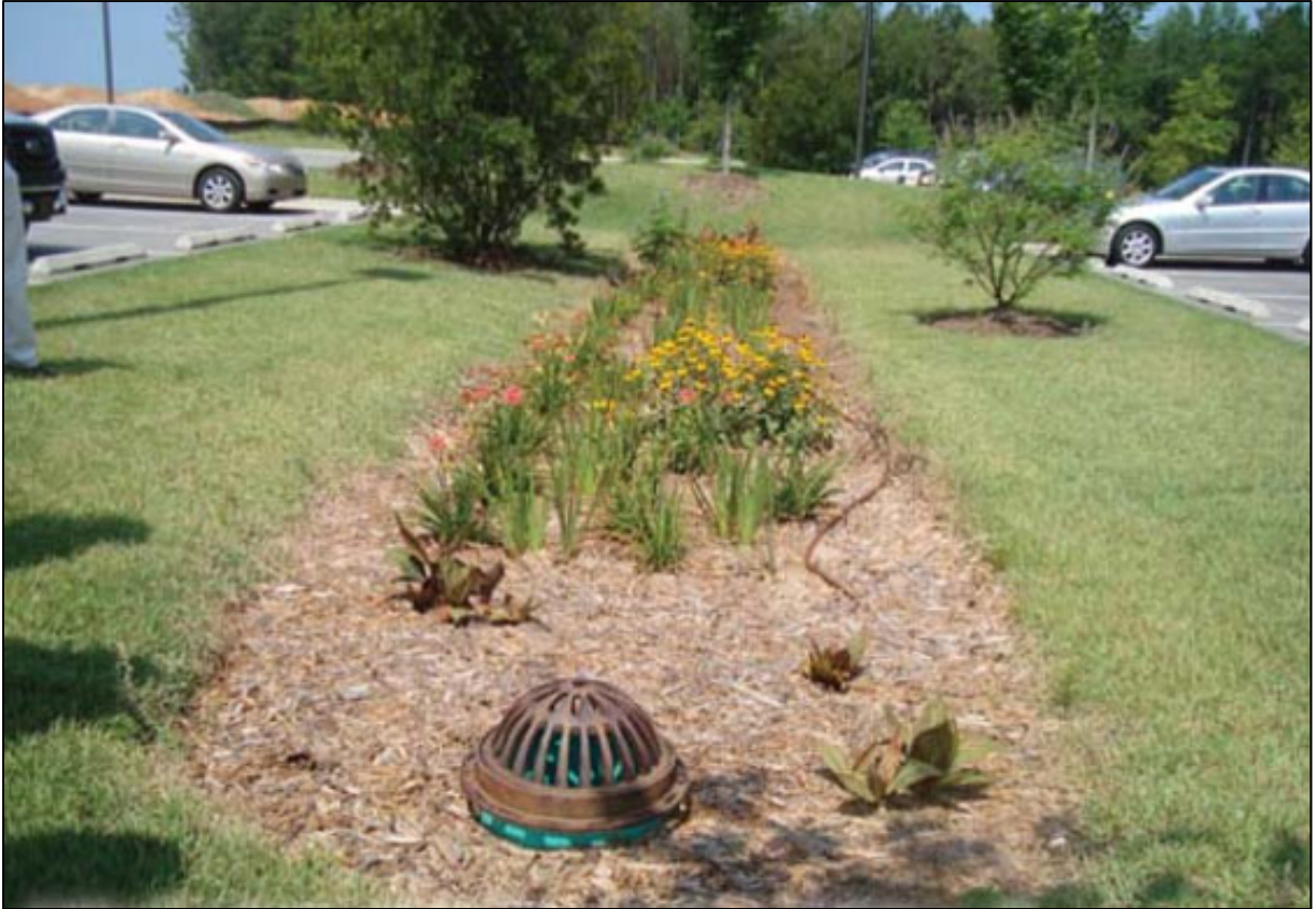
Figure 6.1 Example of bioretention swale in a parking area at Auburn Research Park; Auburn, AL (ADEM 2014)
