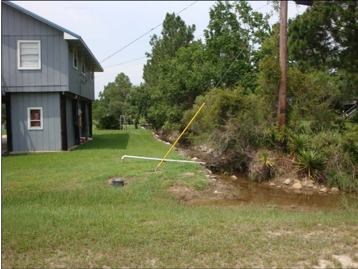
Figure 6.23 Discharge pipe to surface waters of unknown effluent
