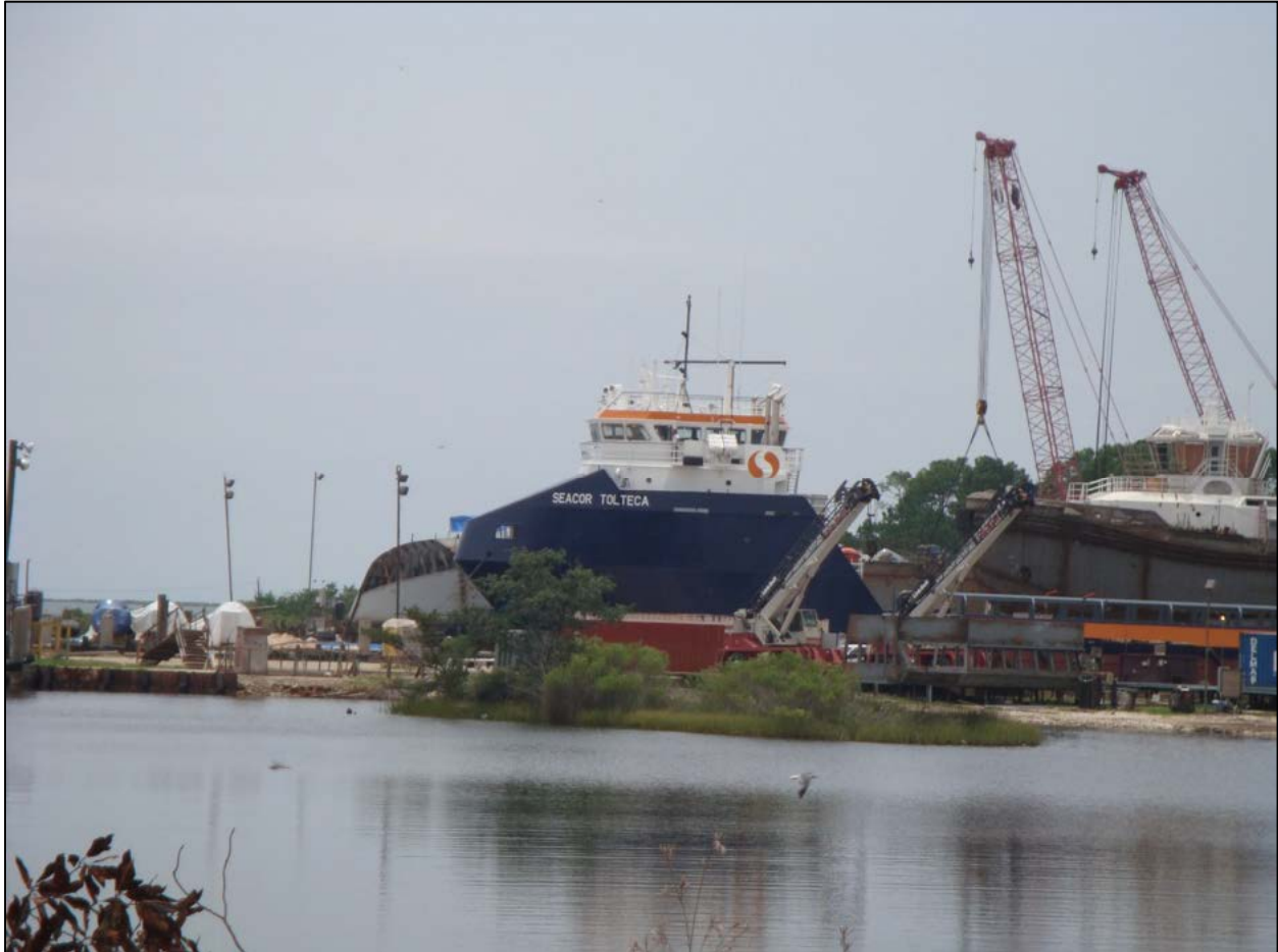
Figure 4.21 Shipbuilding facility on Bayou Coden
