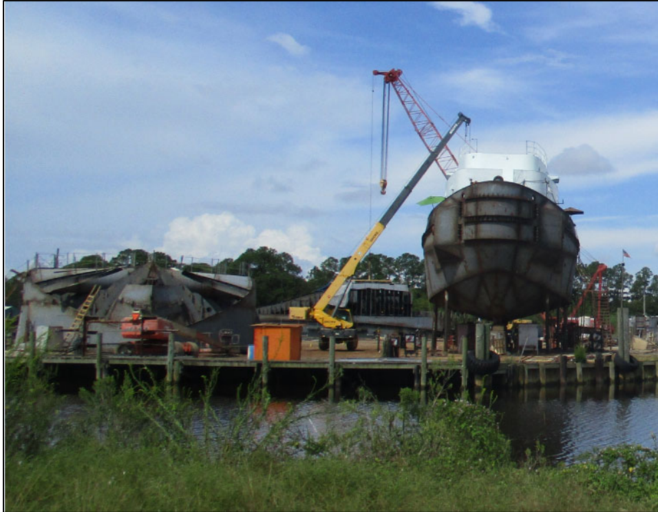
Figure 4.11 Ship repair along the Bayou Coden shoreline
