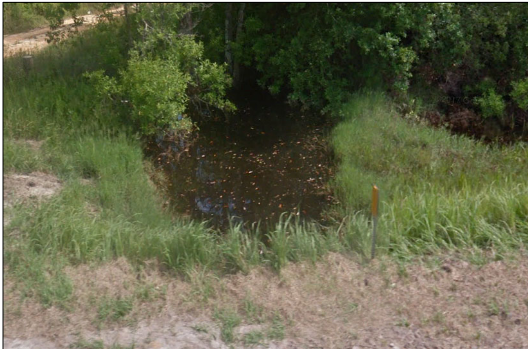
Figure 6.37 Crossing downstream of an unnamed surface water and Highway 188
