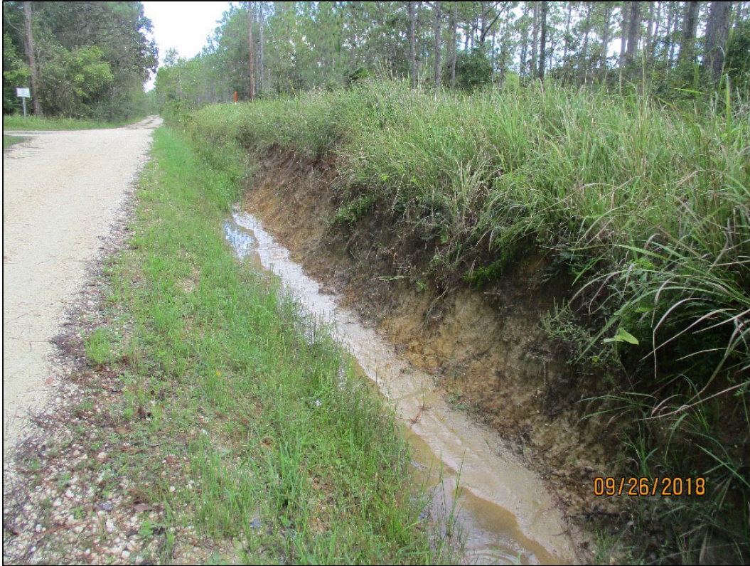
Figure 4.1 Gullying and erosion at Zirlott Road in the eastern Watershed from stormwater runoff
