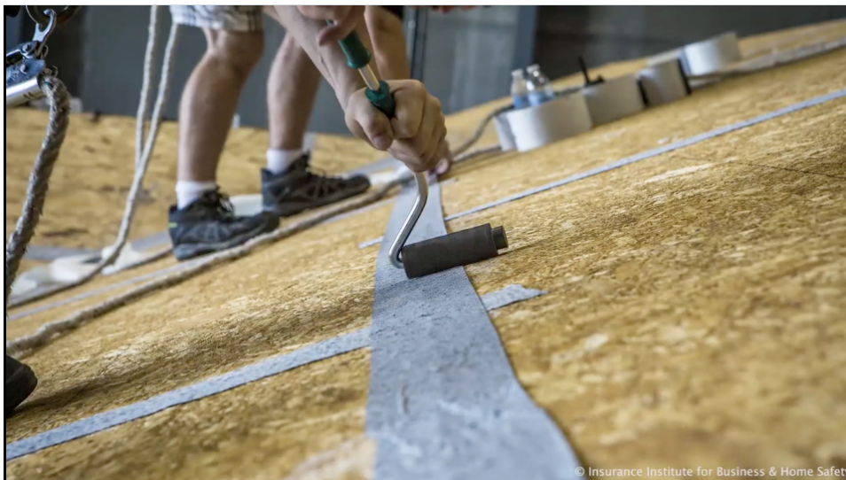
Figure 3. Installing a sealed roof deck system; taping the seams of roof sheathing.
