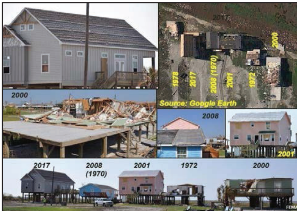
Figure 71 Willacy County, Texas (Demonstrating how different building codes fair during a storm)
