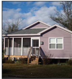
Pier foundation with crawlspace
