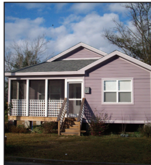
Pier foundation with crawlspace
